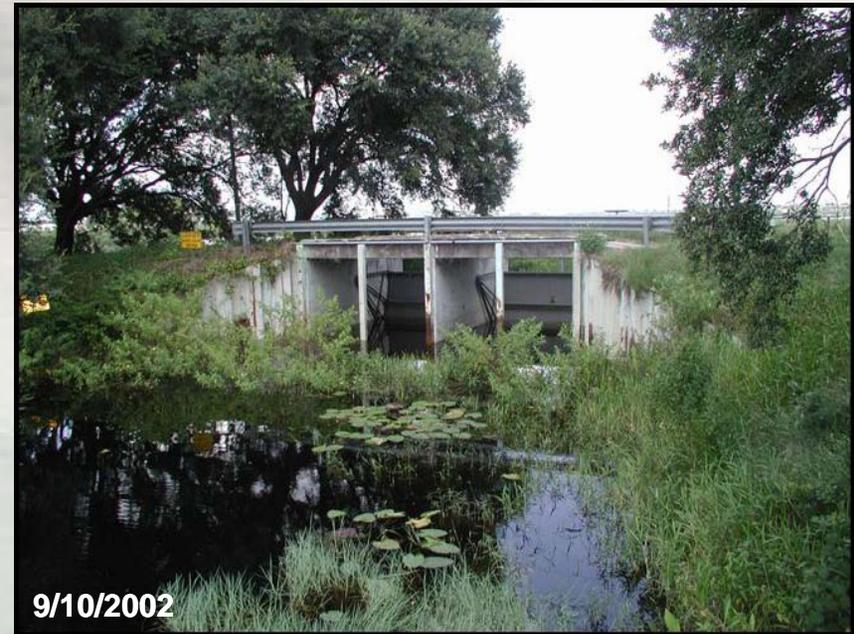
**Note:** Downstream lake level was higher than upstream lake level on September 10, 2002. A foot to a foot-and-a-half of water was being retained above the base of the structure on the downstream side.
