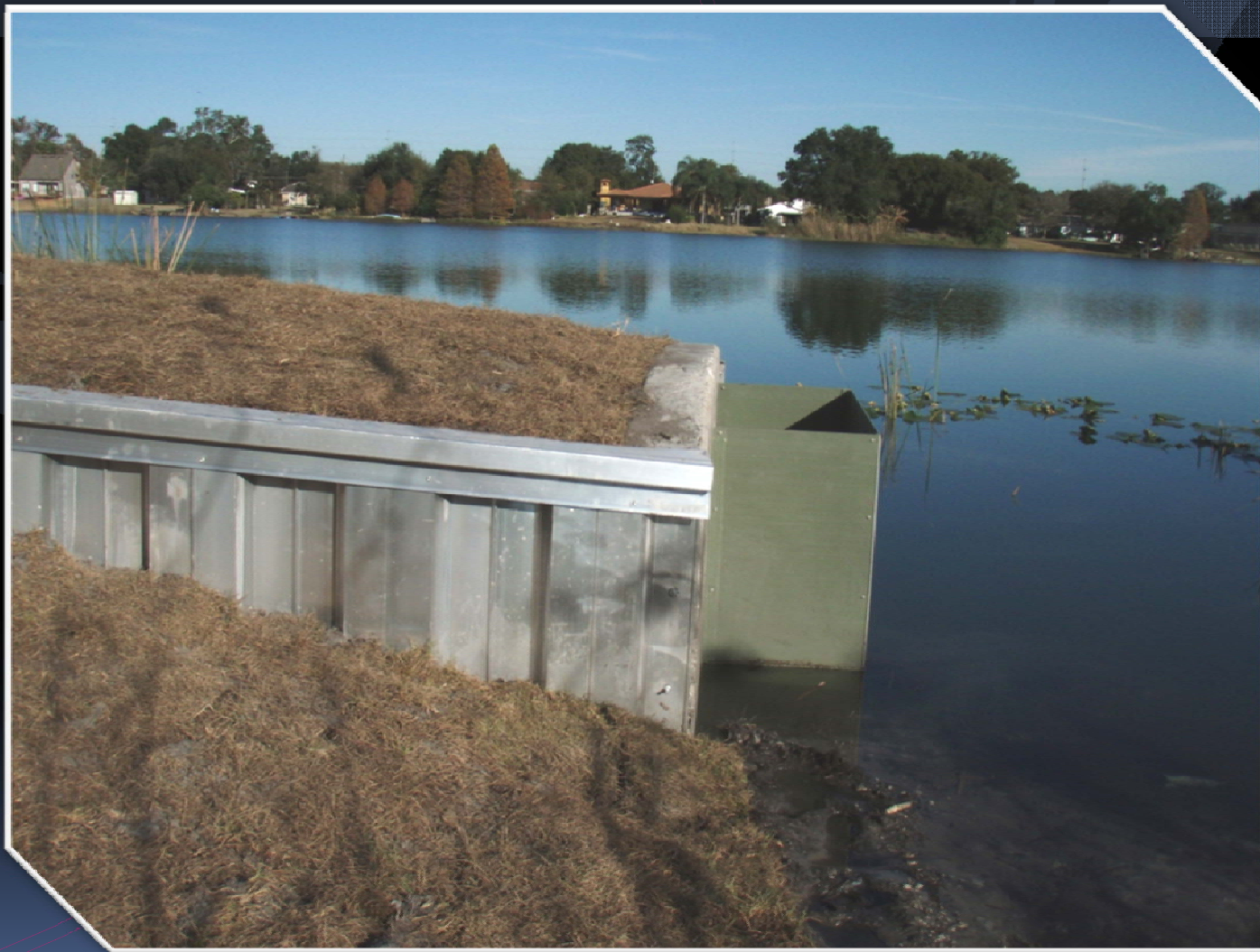
Bass Lake - Complete sheetpile wall with end wall and skimmer
