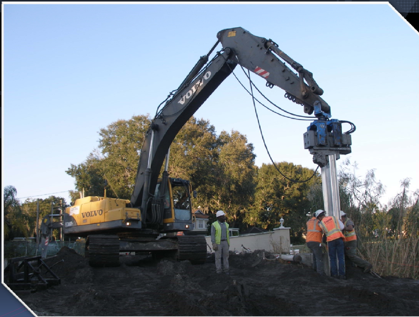
Bass Lake - View of trackhoe-mounted hammer during sheet pile wall installation.
