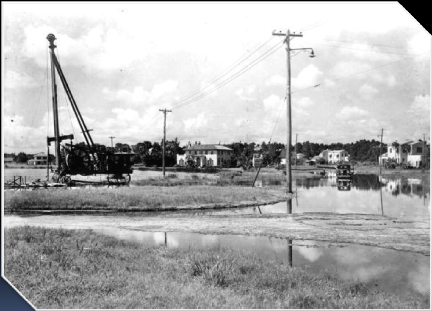
Rig in photograph was used to drill deeper drainage well
