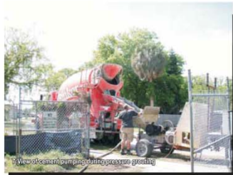
7-View of cement pump during grout injection
