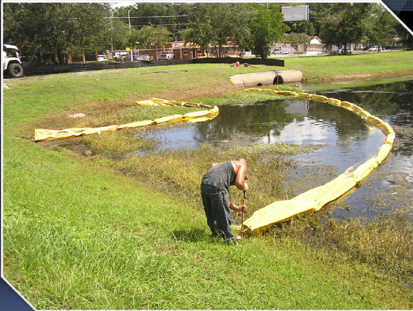
Bumby Avenue - Turbidity barriers being set up prior to construction activities.
