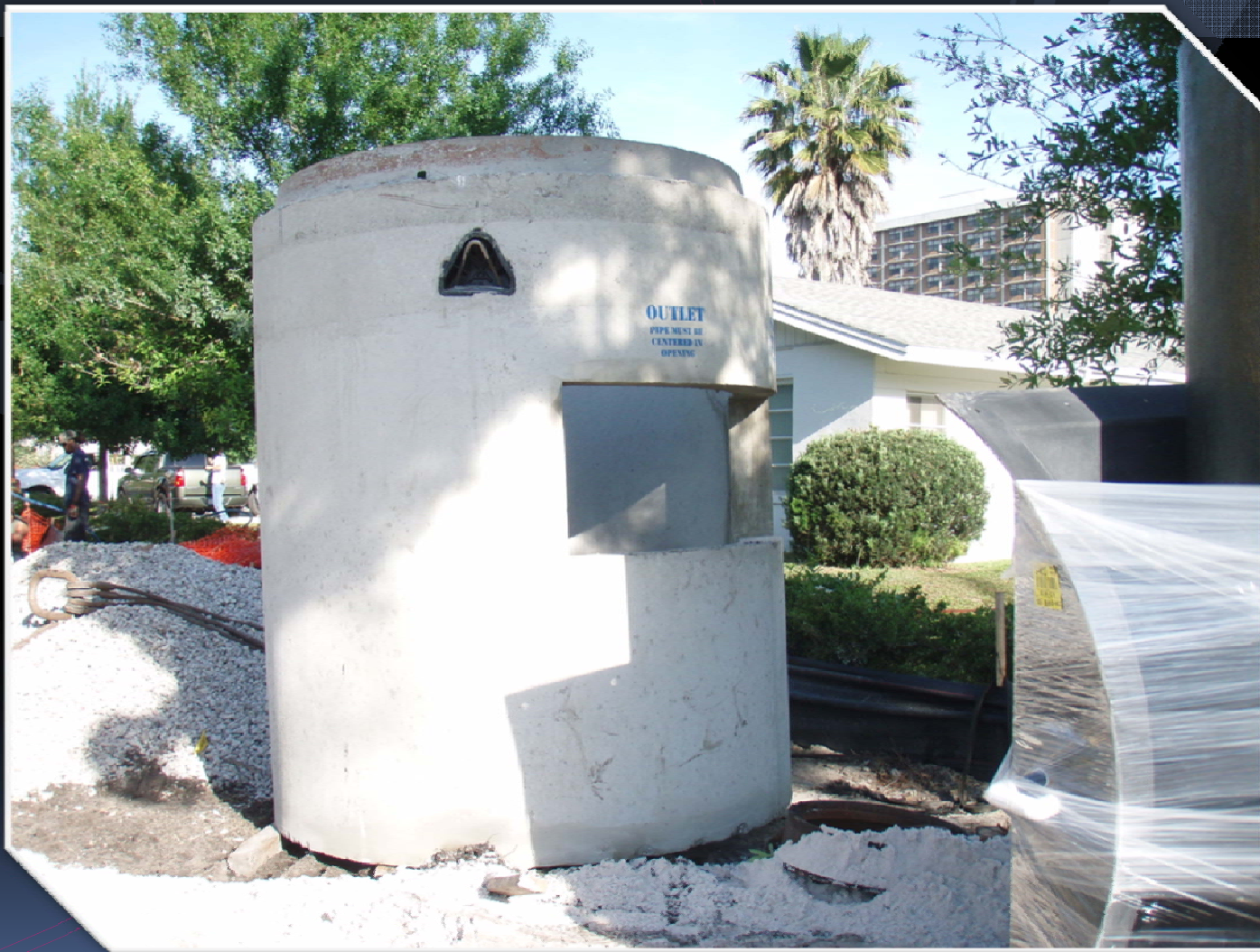
Clay Street - CDS stormwater treatment unit prior to installation.
