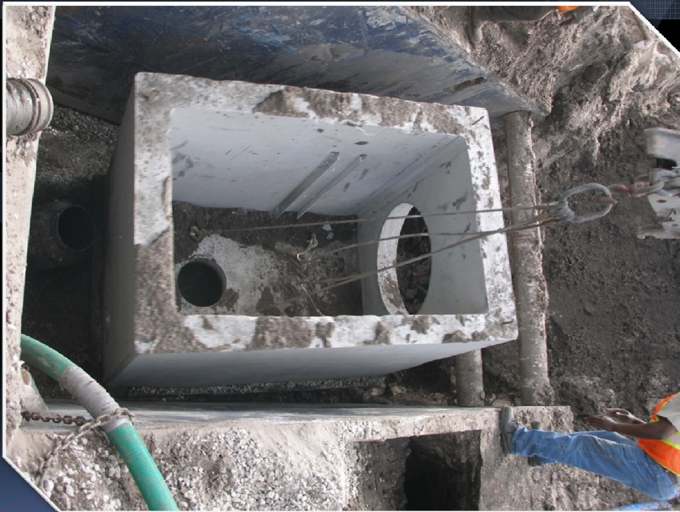
Bass Lake - View of enclosure being installed.
