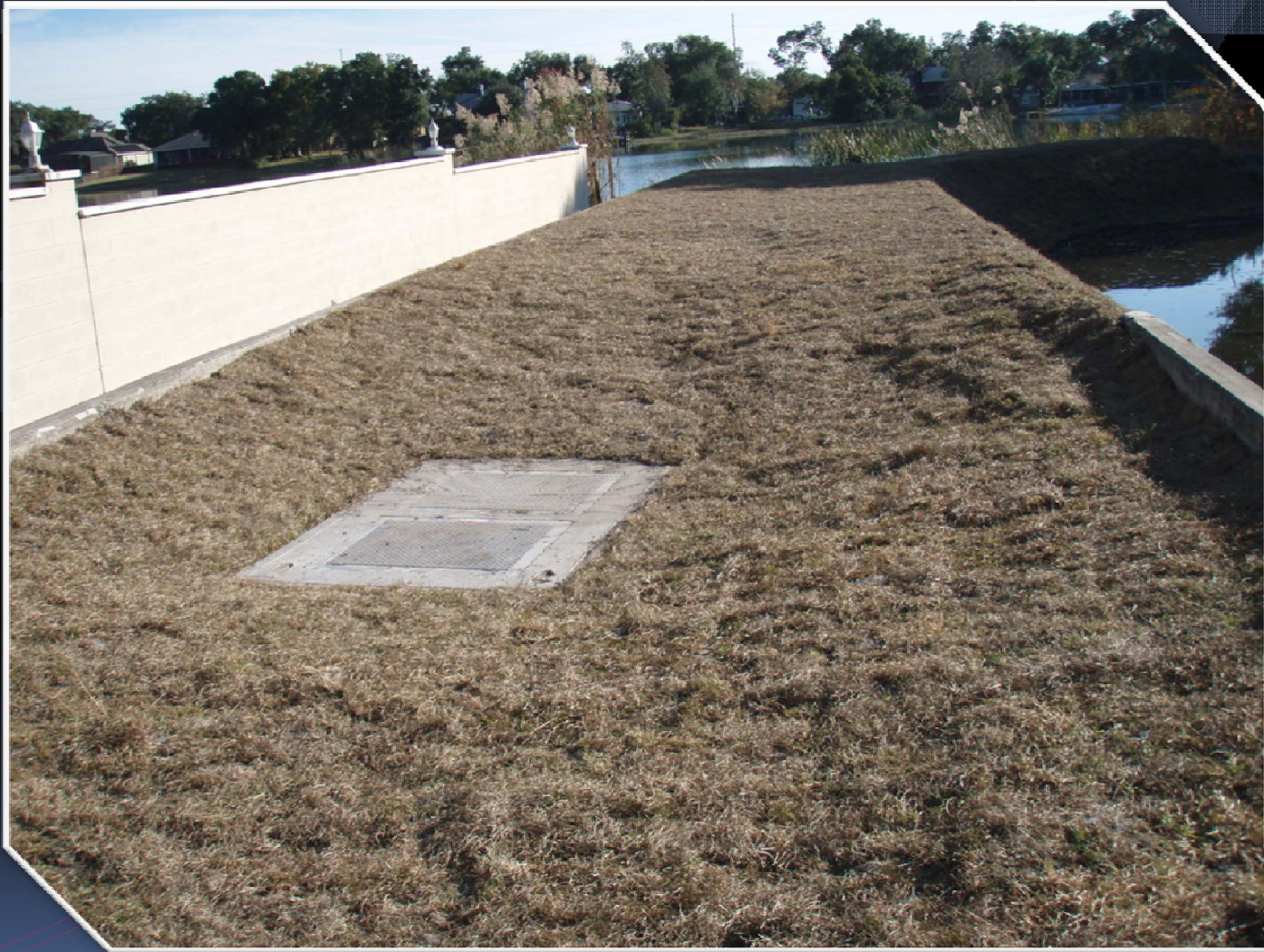
Bass Lake - View showing enclosure with aluminum hatch at new well.
