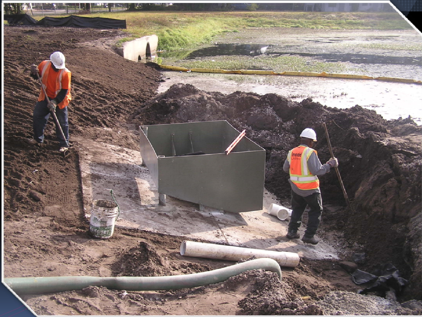
Bumby Avenue - Fiberglass skimmer being set into position on inflow structure.
