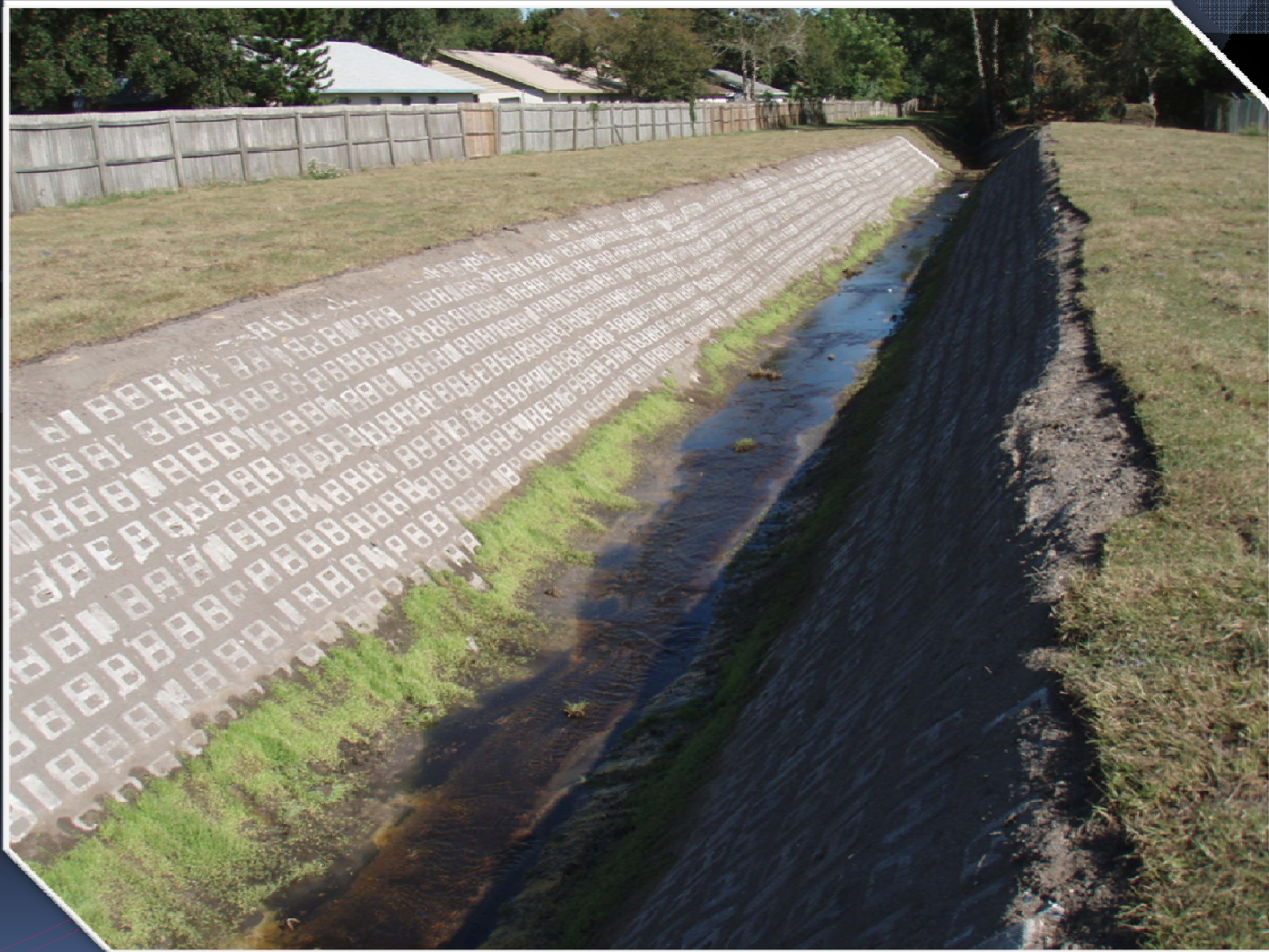
Goddard Avenue - Cable concrete ditch enhancement installed by Orange County personnel.
