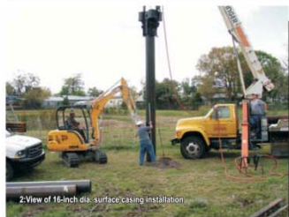
2-View of 16-inch dia. surface casing installation
