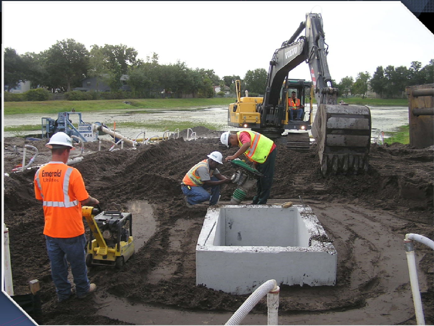
Bumby Avenue - Backfilling and compacting area around new well enclosure.
