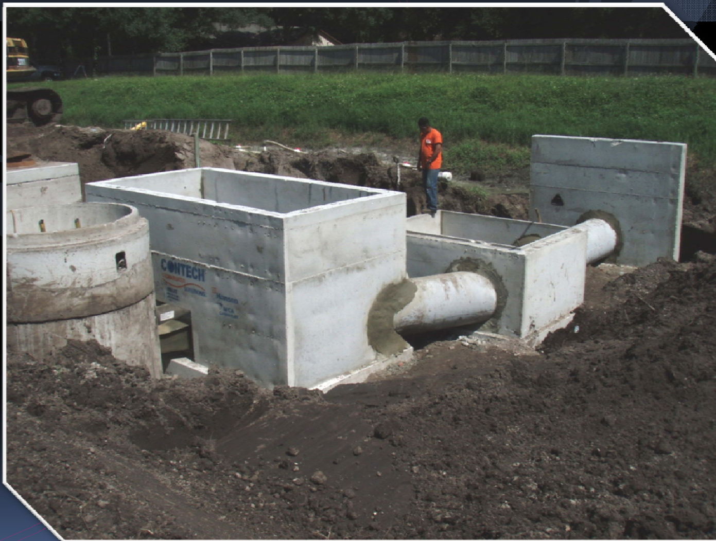
Goddard Avenue - Structure and pipe installations prior to backfilling.
