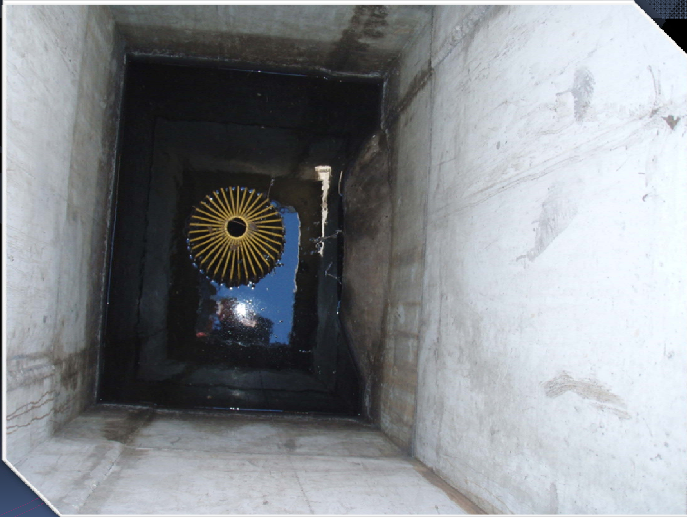
Goddard Avenue - Interior of DW-031 well structure.
