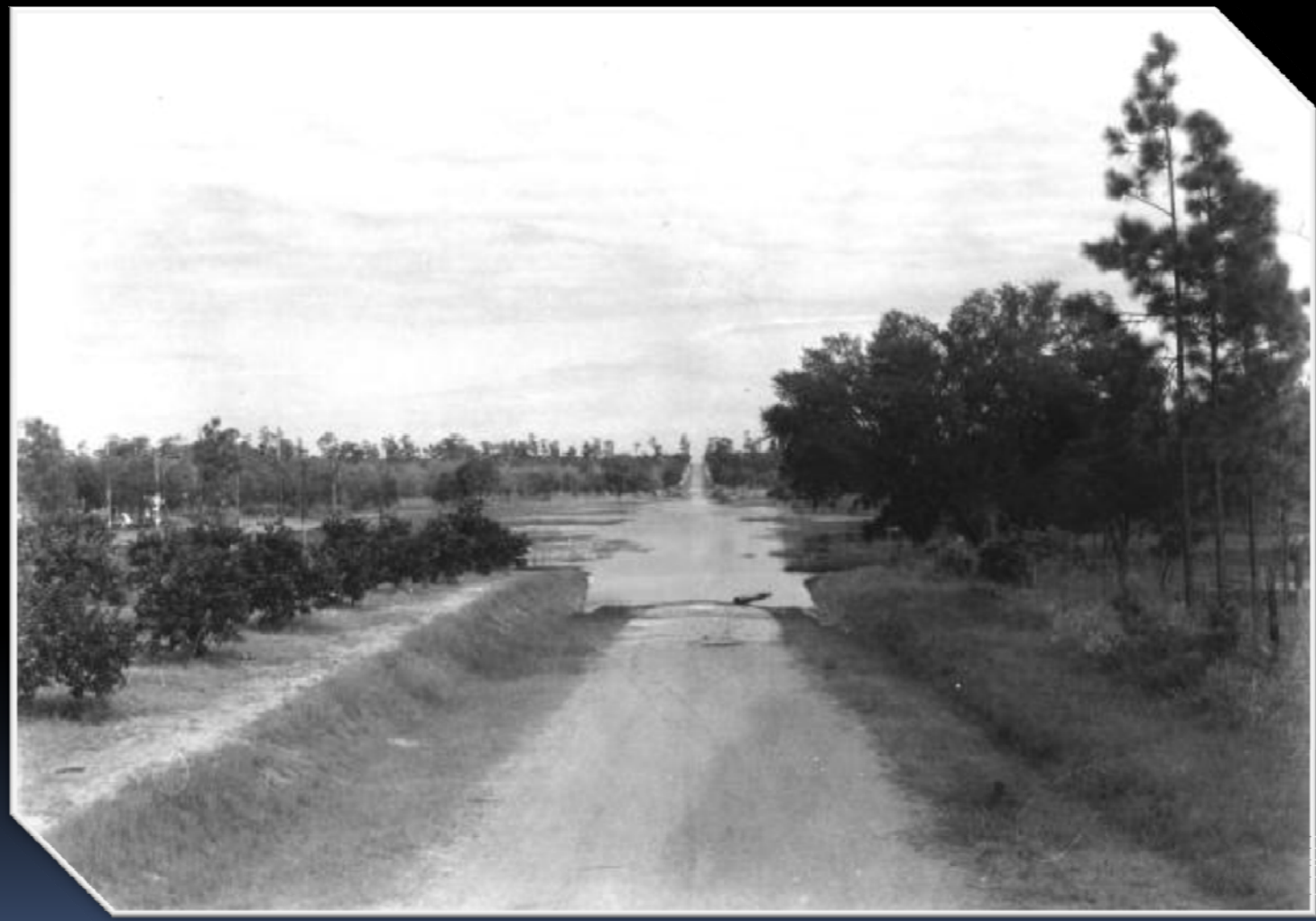
This photo was taken before Hiawassee Rd was realigned
