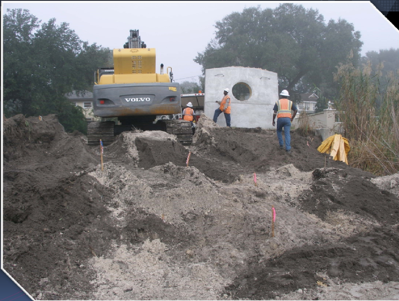
Bass Lake - View of headwall during installation activities.
