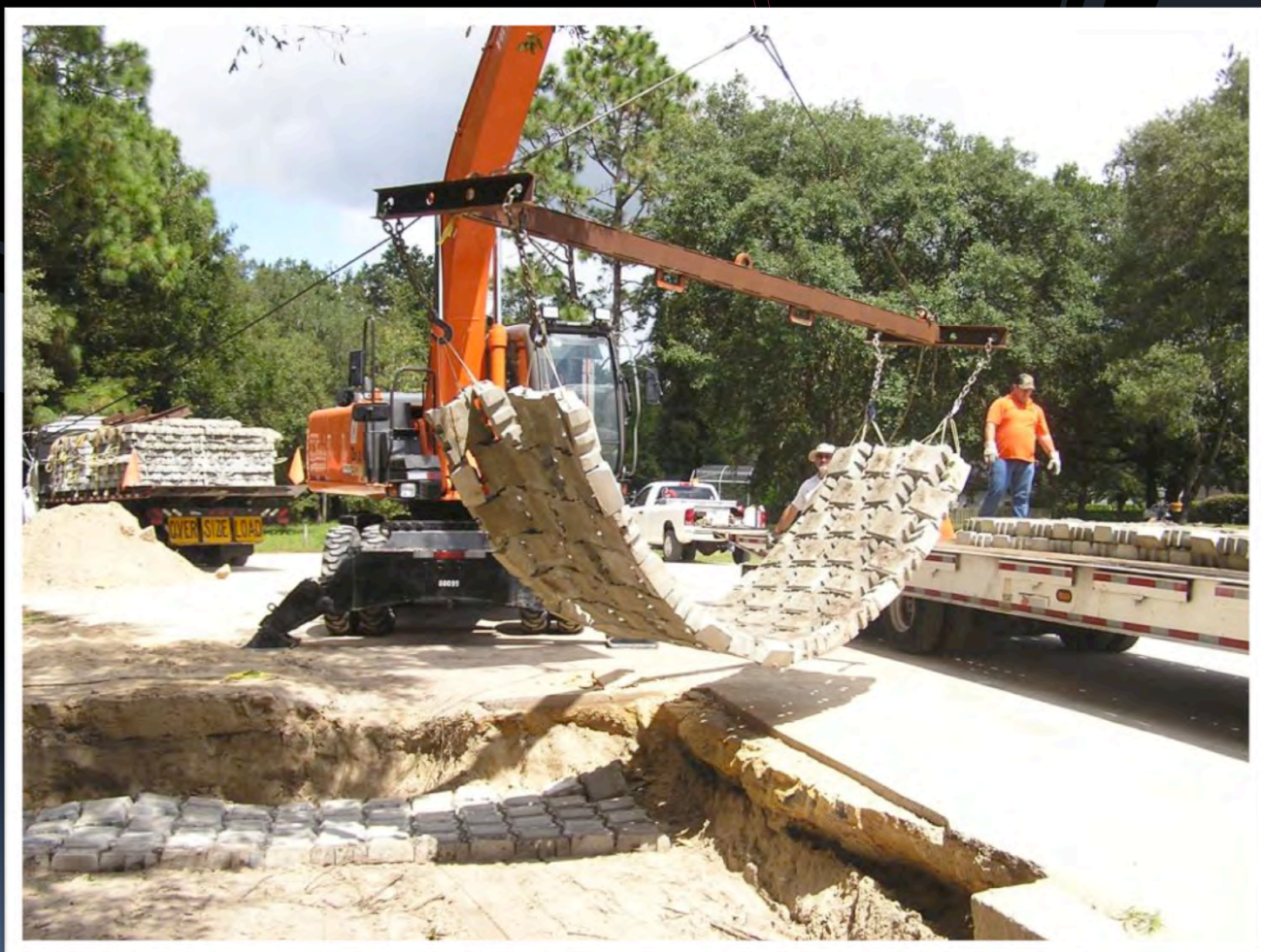
Cable concrete being placed into position (Sep 23)
