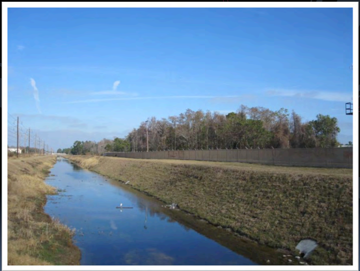
Completion Photo 6 months after construction
