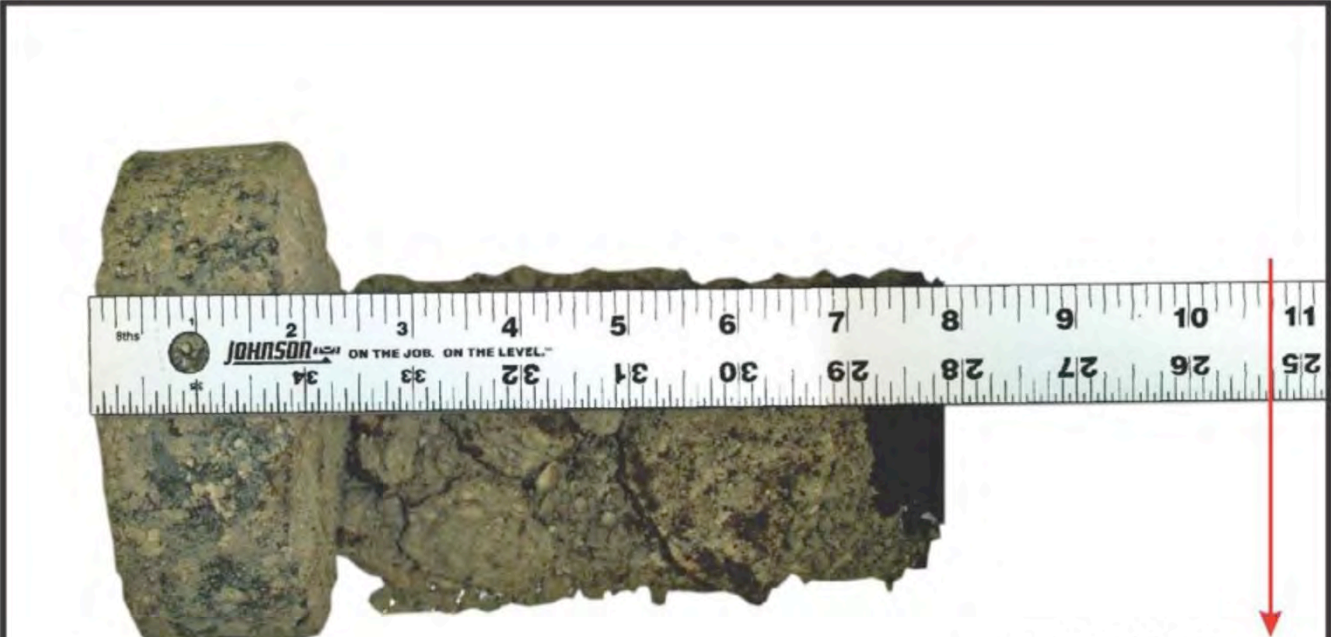
Approx. depth to bottom of base course as measured in corehole.
