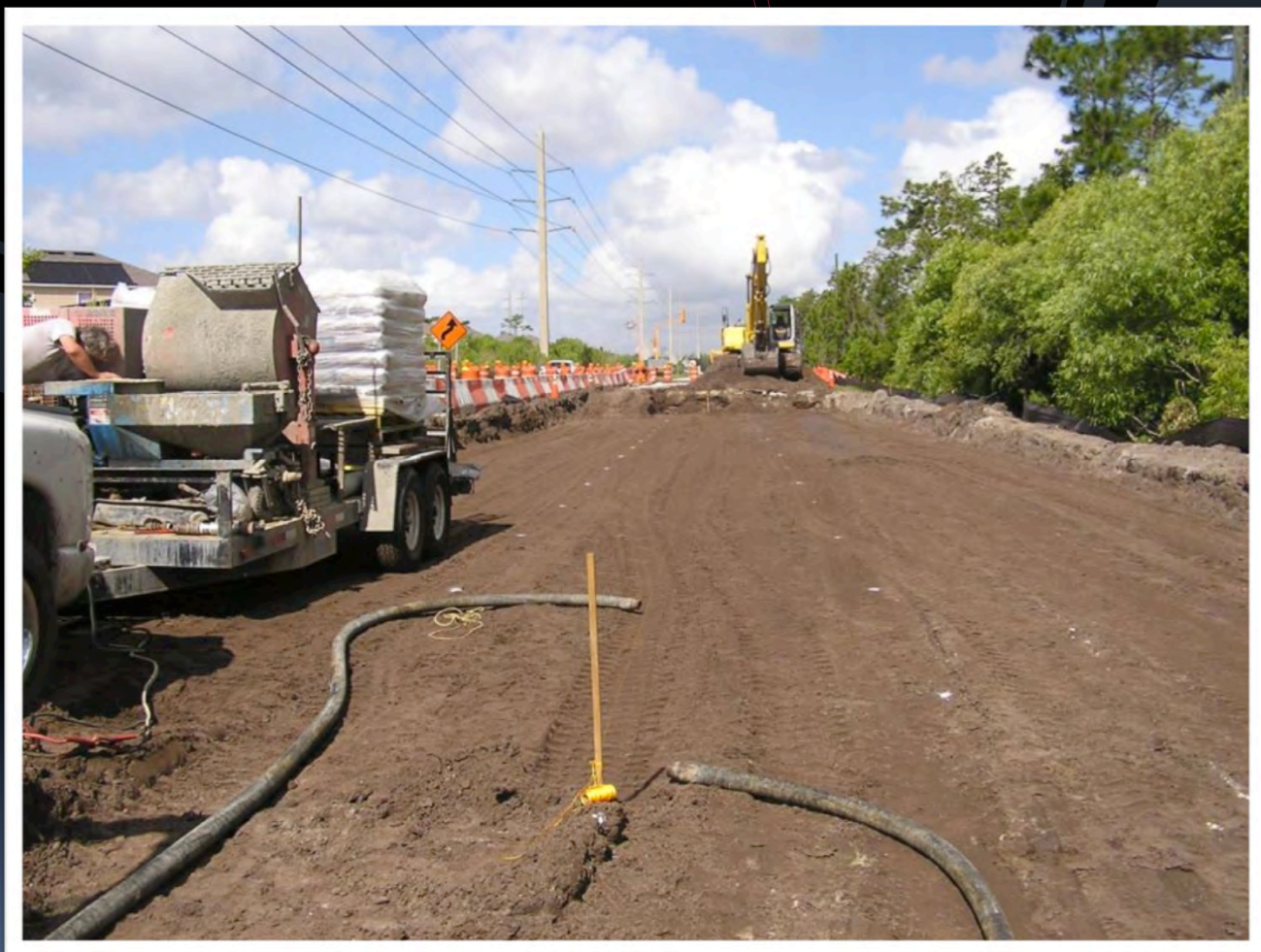
Grout injection on April 24, 2008
