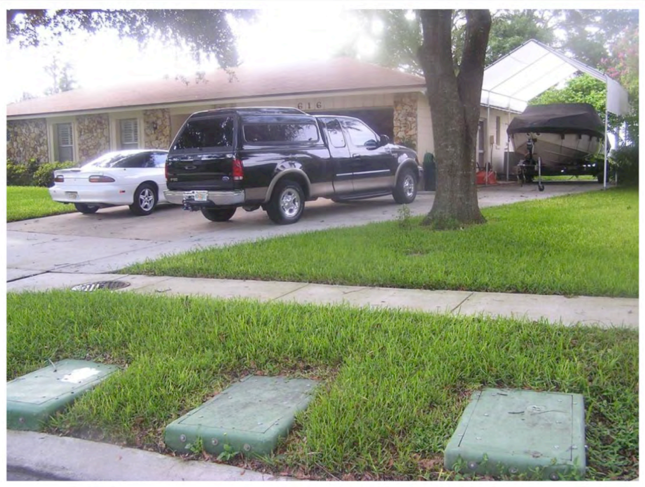
Installed structure in landscape strip
