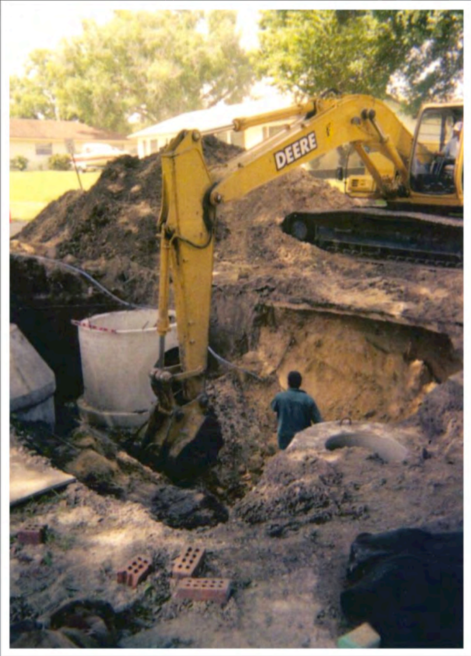
Photos of installation
