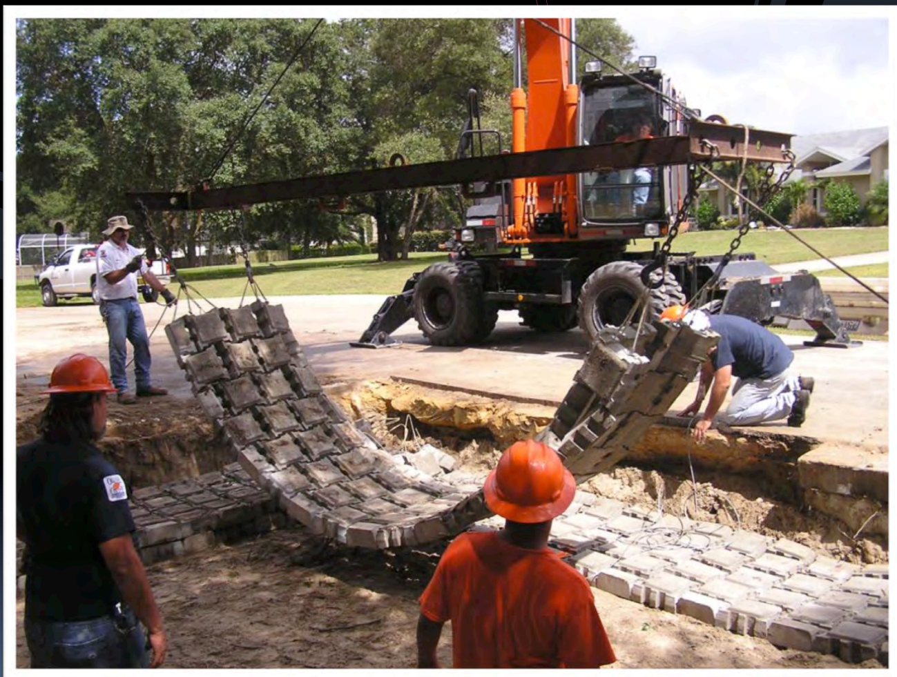
Another panel being placed (Sep 23)
