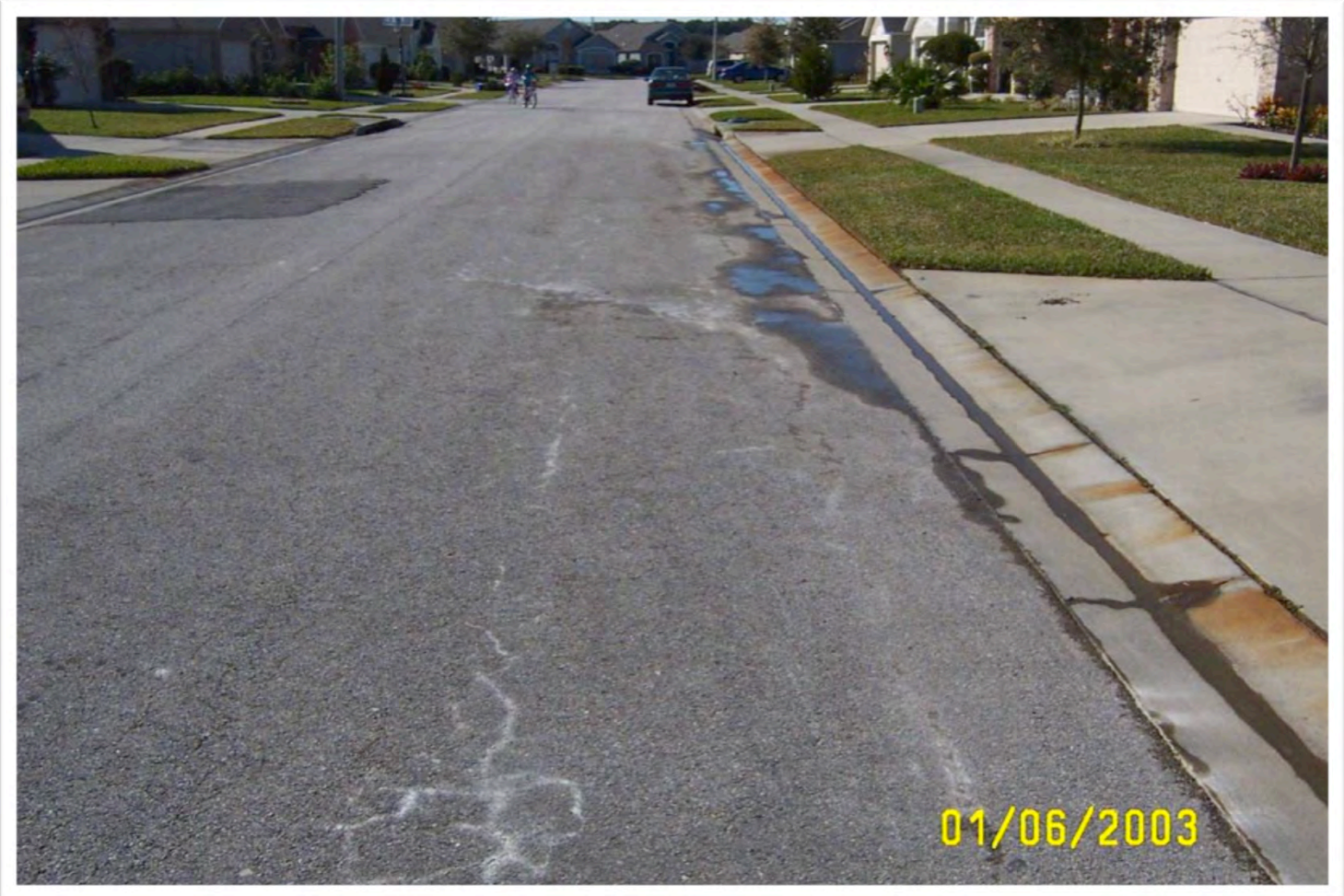
Limerock Pumping From Base
