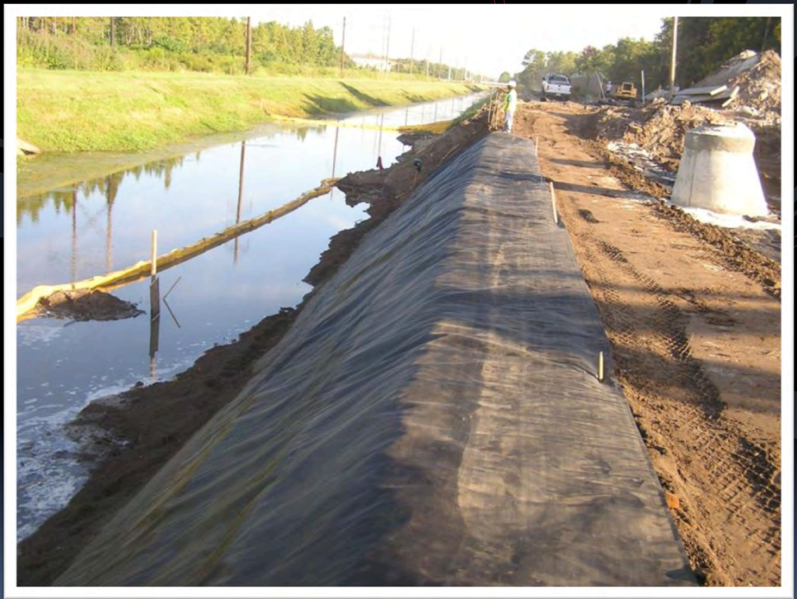
Slope Work Nearing Completion
