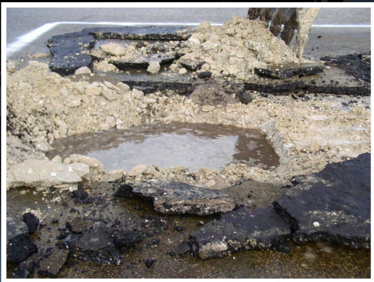
Field Investigation and Excavation
