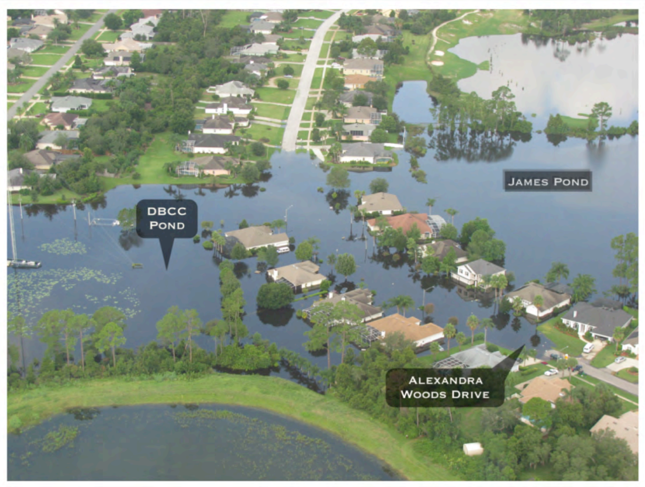
James Pond (9 structures flooded)
