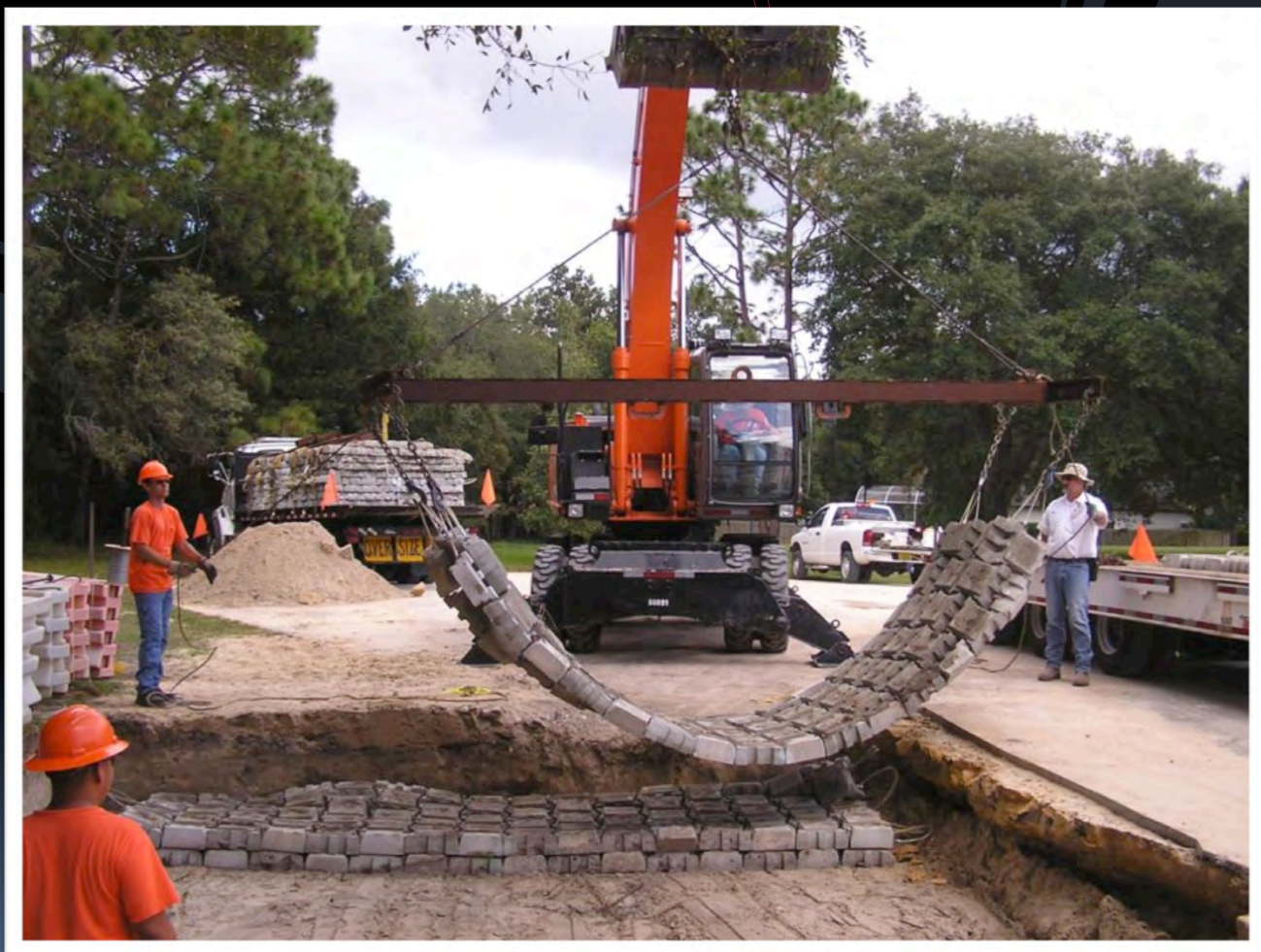
Cable concrete being guided into position (Sep 23)
