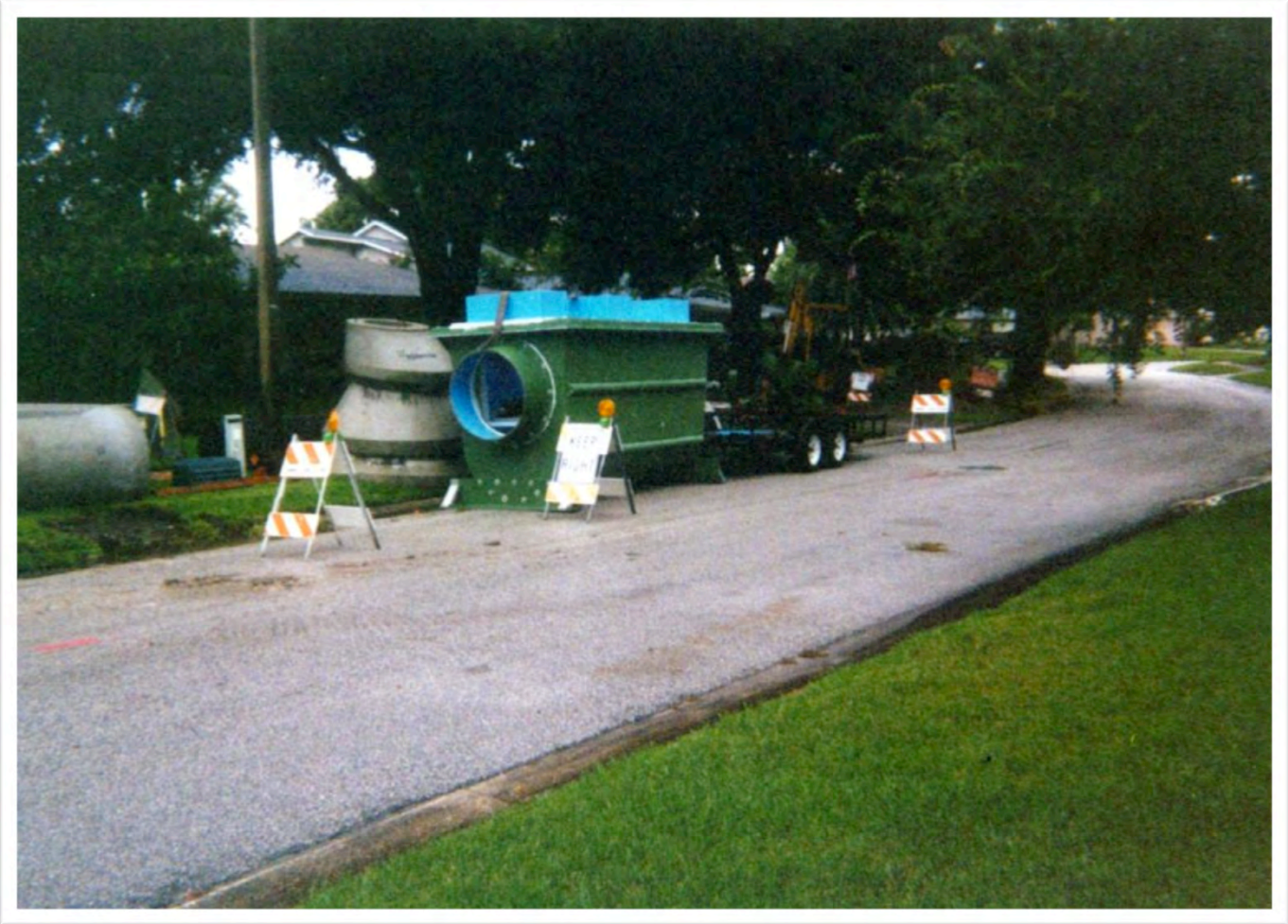
Photos of installation
