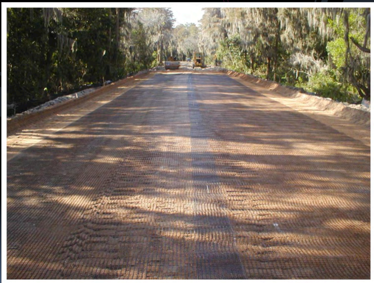
Geogrid installation during repair
