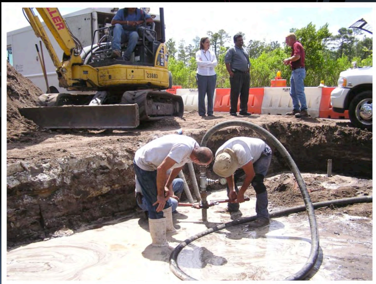
Another grout injection on April 24, 2008
