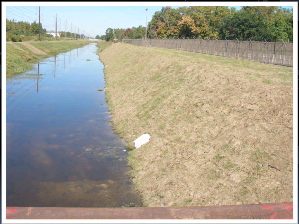
Slope Upon Completion
