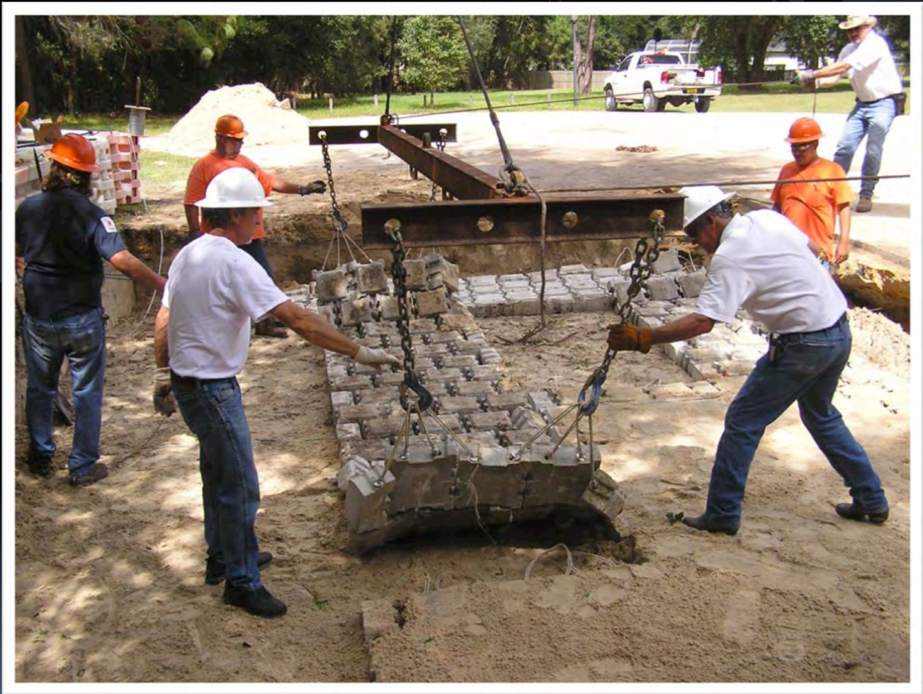
Panel being positioned by county staff (Sep 23)
