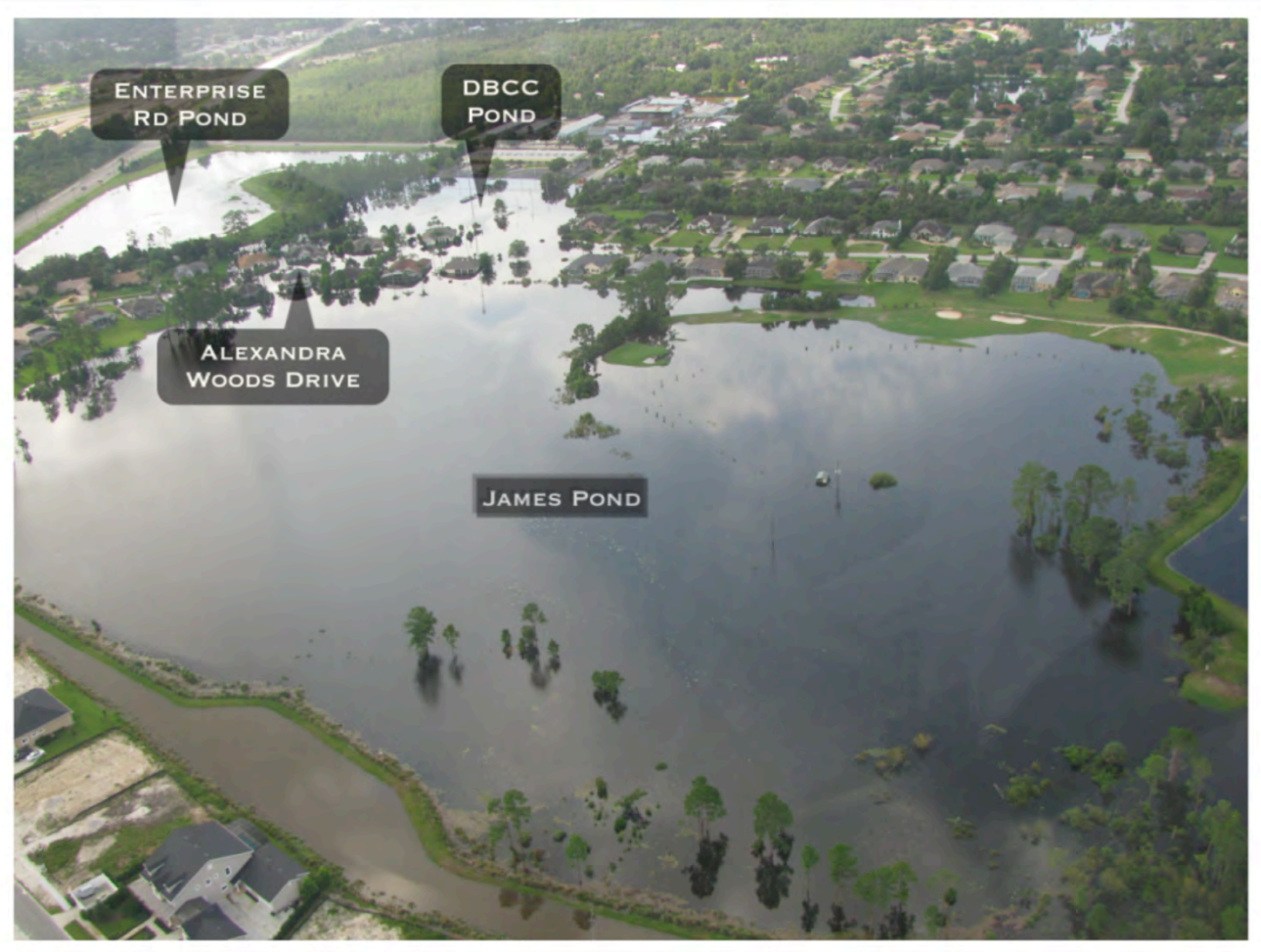
James Pond (9 structures flooded)
