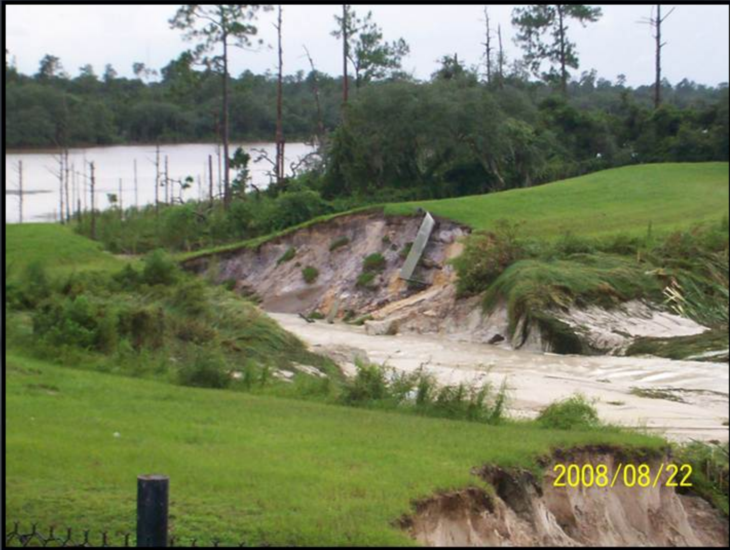
Miller Road Pond Outfall (Photo 1 of 4)
