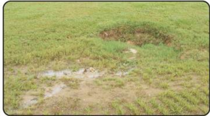
Photo 2. Shows Water Flowing into The Sinkhole at the Toe of Slope on the Western Side of Pond SMF-1 on October 24, 2007
