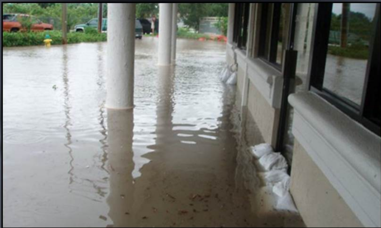
Flooding at Downstream Building
