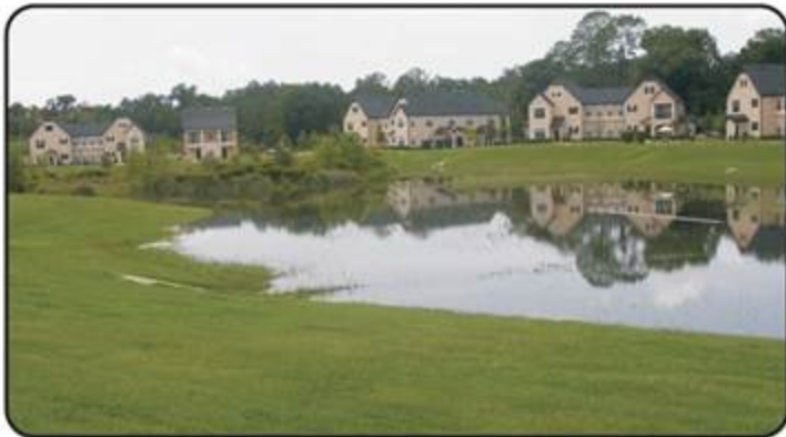
Photo 3. Shows Pond SMF-1 at its Highest Stage on July 9, 2008
