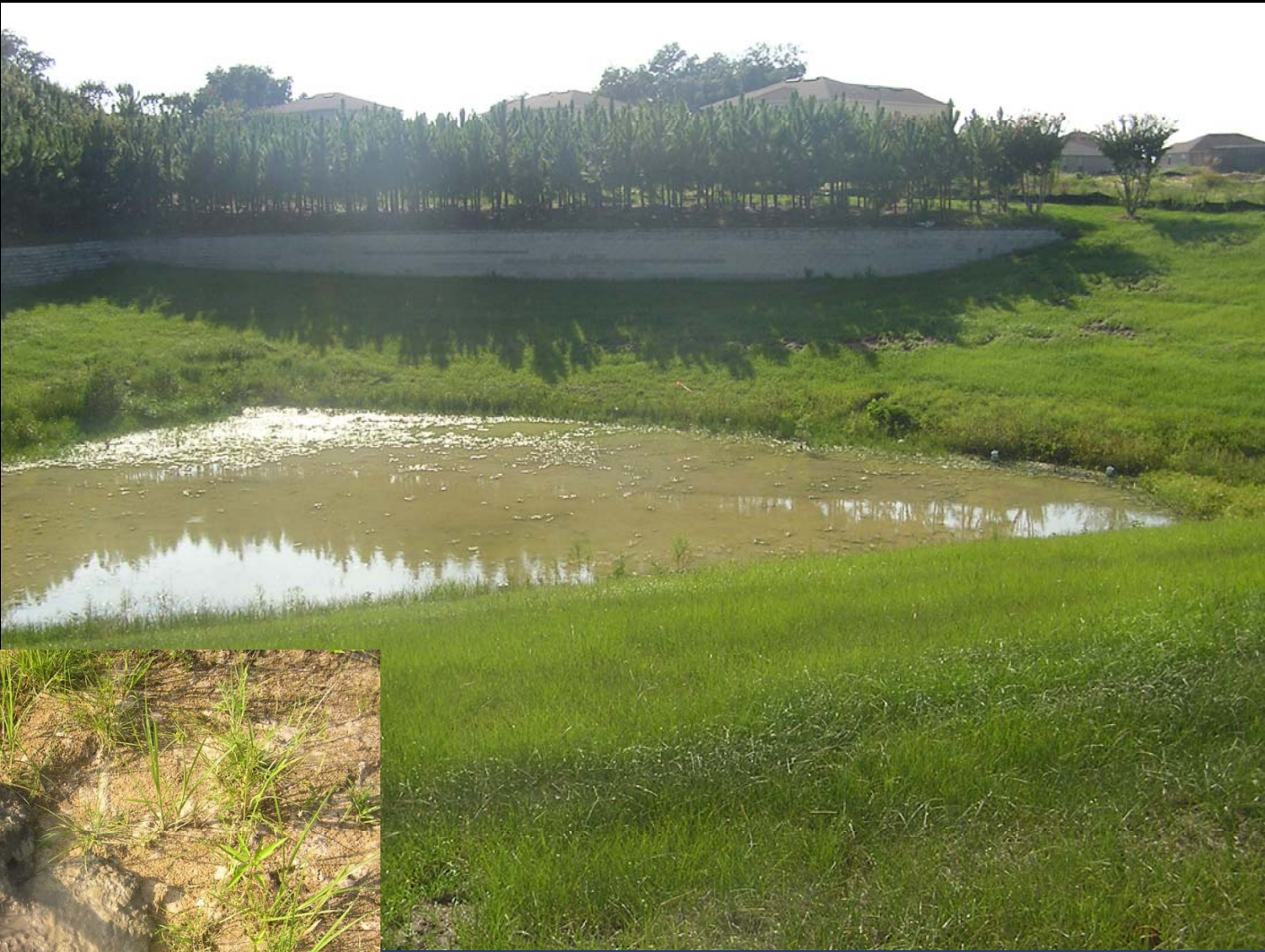
Standing water in pond after installation of underdrains
