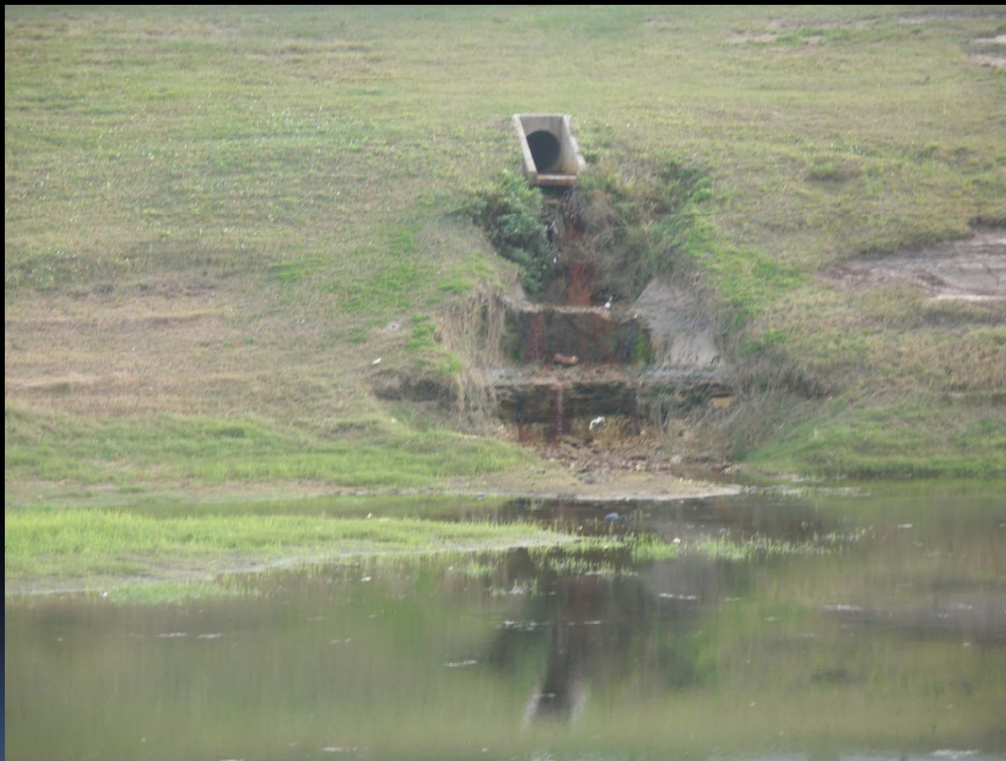
WESTLAKE-Resulting Cascading Outfall to Pond
