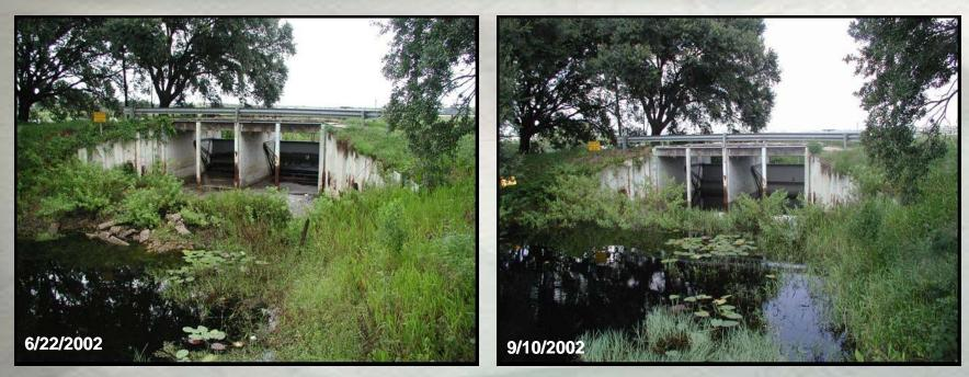
**Note:** Downstream lake level was higher than upstream lake level on September 10, 2002. A foot to a foot-and-a-half of water was being retained above the base of the structure on the downstream side.
