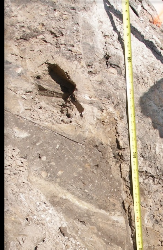
Close-up view of the shear failure plane on the northern pit wall
