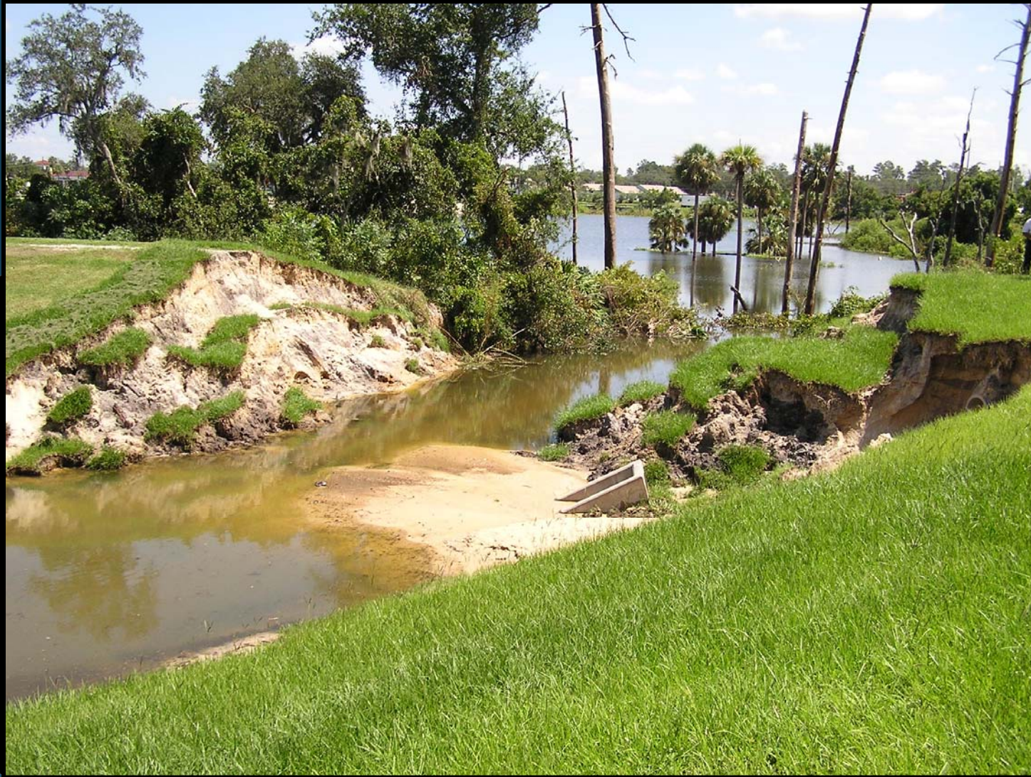
Grande Ville Apartments (Photo 3 of 4)
