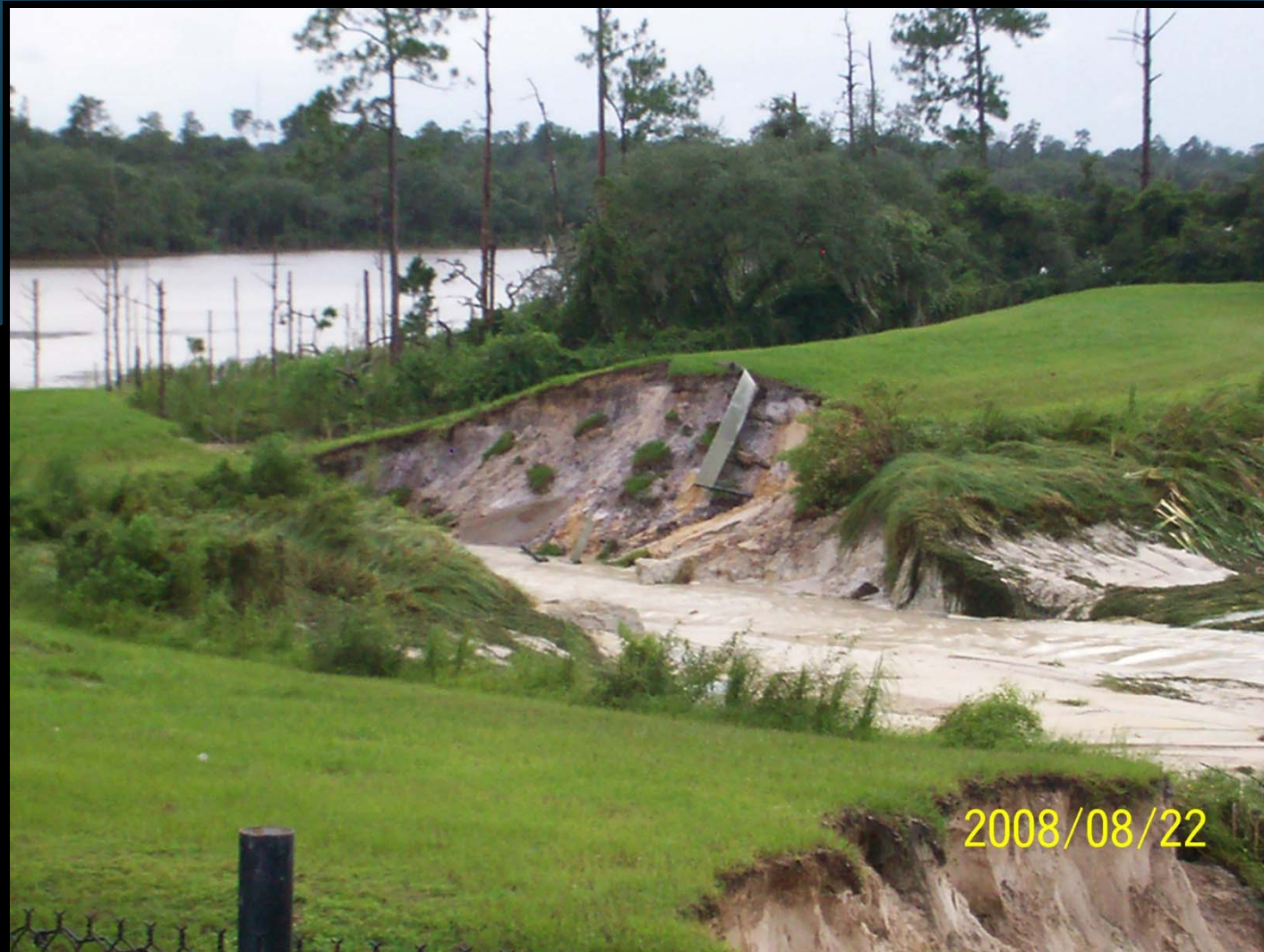
Miller Road Pond Outfall (Photo 1 of 4)
