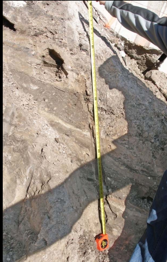
View looking at the shear failure plane on the northern pit wall
