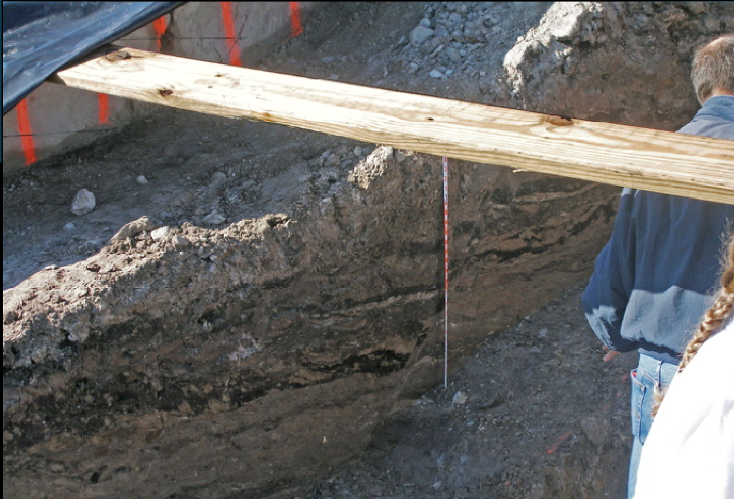
Example of Test Pit Showing Shear Plane
