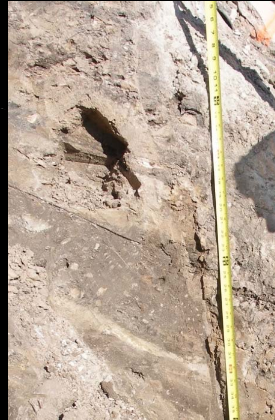
Close-up view of the shear failure plane on the northern pit wall
