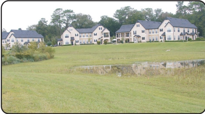
Photo 1. Shows Some Standing Water in Pond SMF-1 on October 24, 2007
