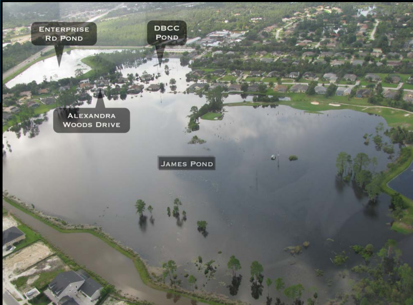
Highbanks Enterprise Road Pond James Pond (9 structures flooded)
