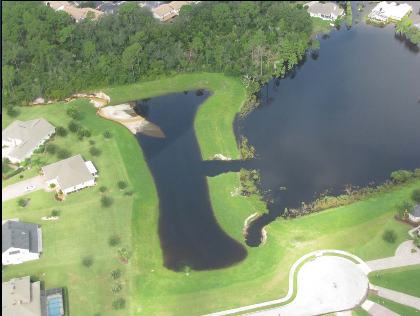
Glen Club Drive Pond Berm Failure (Photo 2 of 4)
