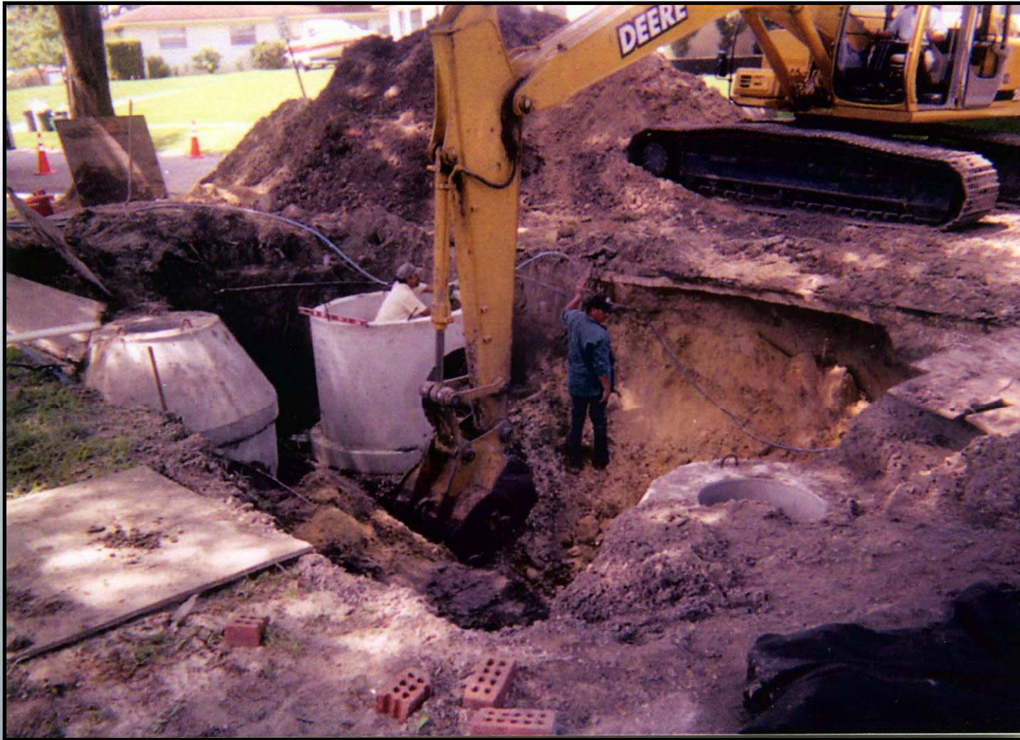
Photos of installation
