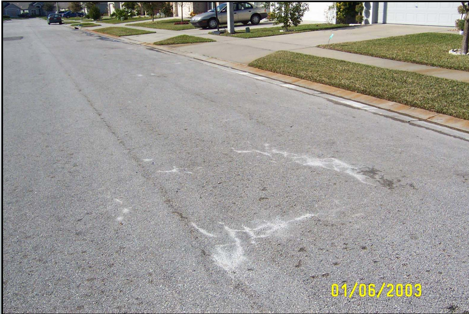
Limerock Pumping From Base
