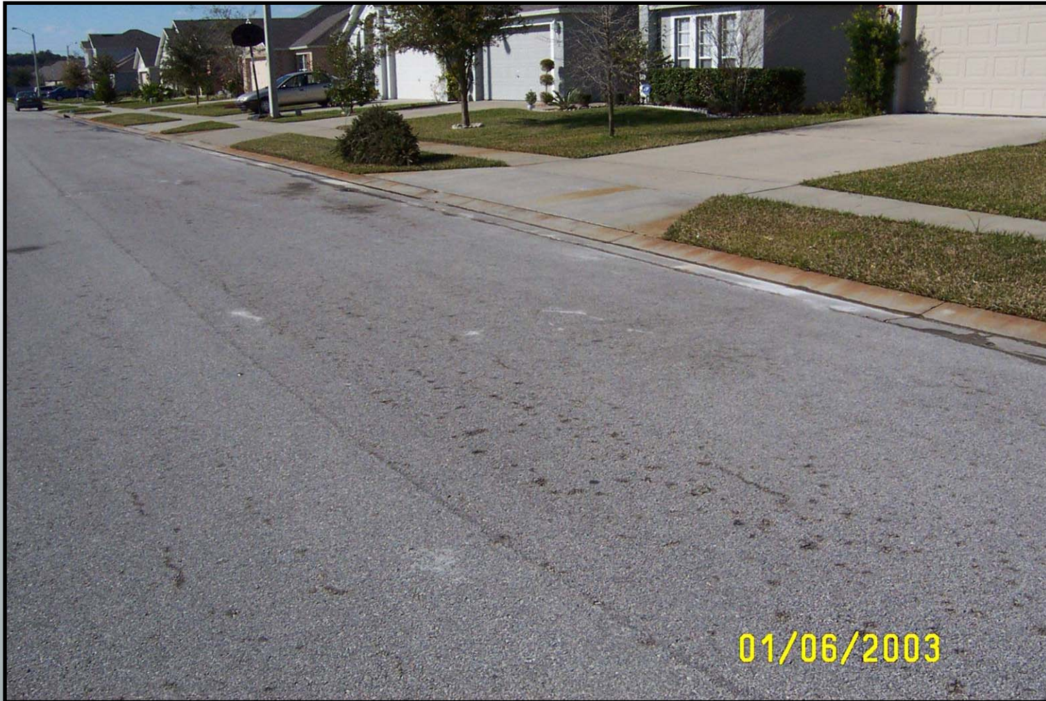
Leaching Over Curb
