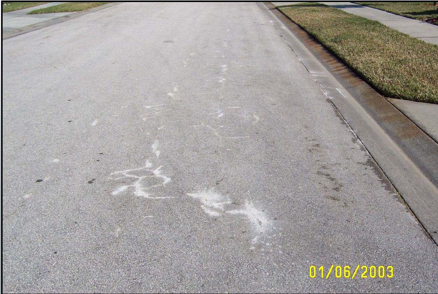
Limerock Pumping From Base
