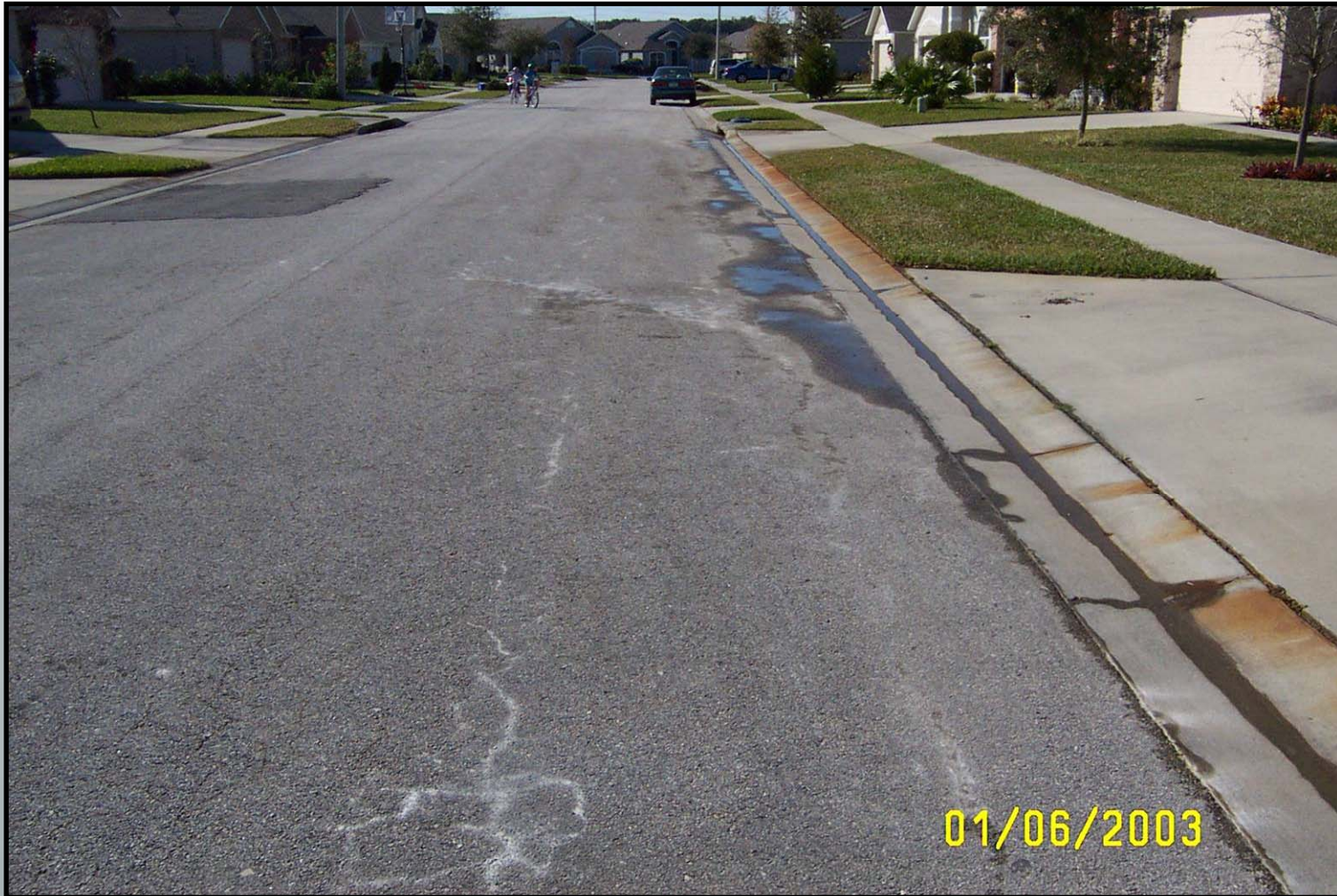
Limerock Pumping From Base
