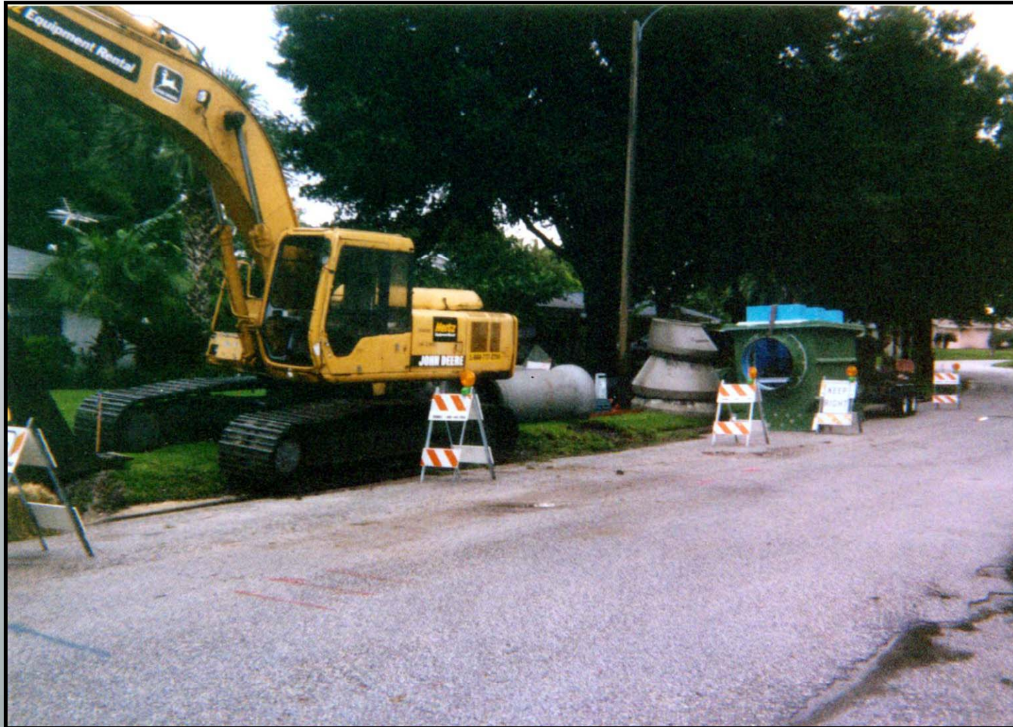
Photos of installation
