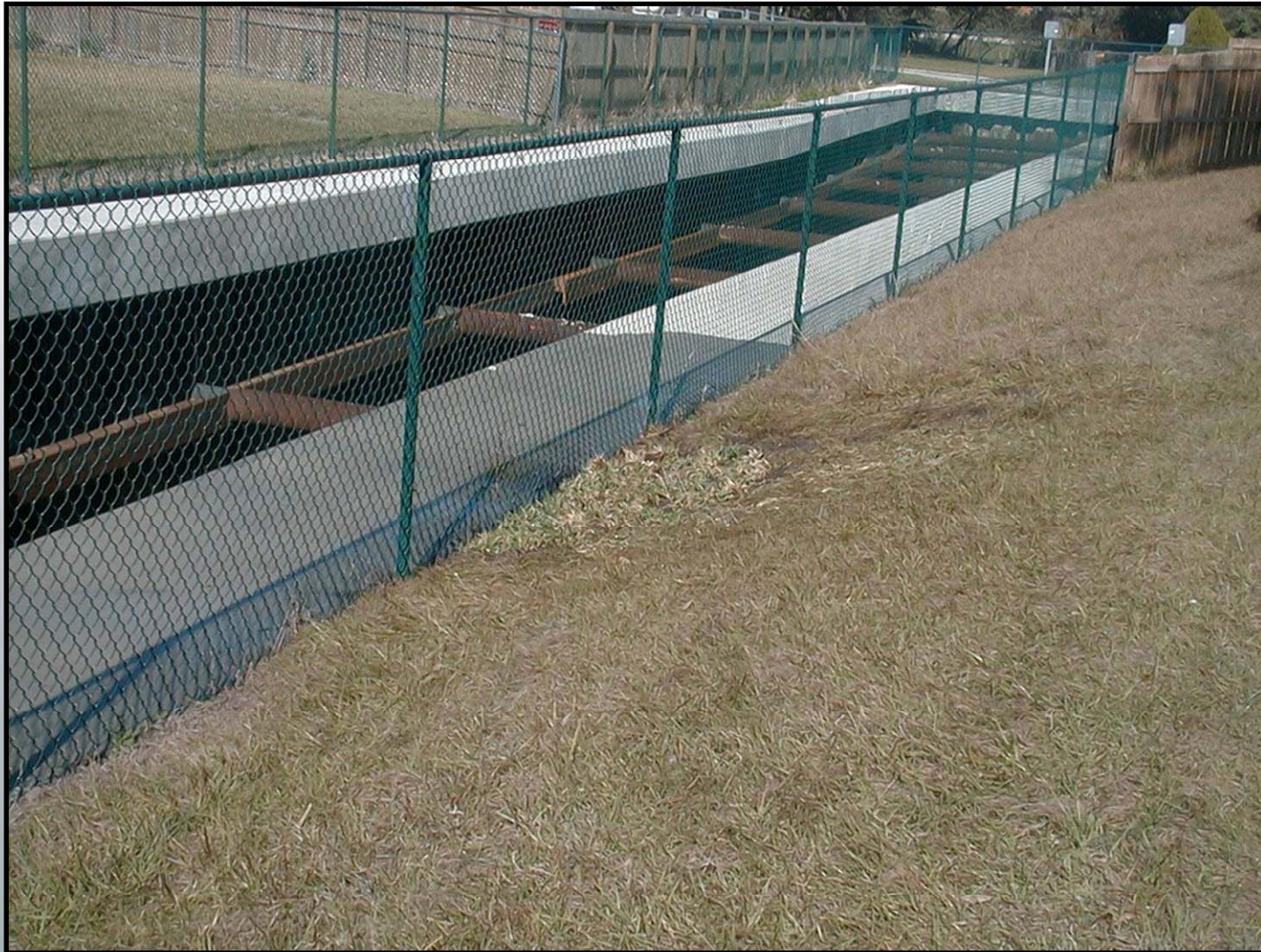
View of depression area after grouting, facing north
