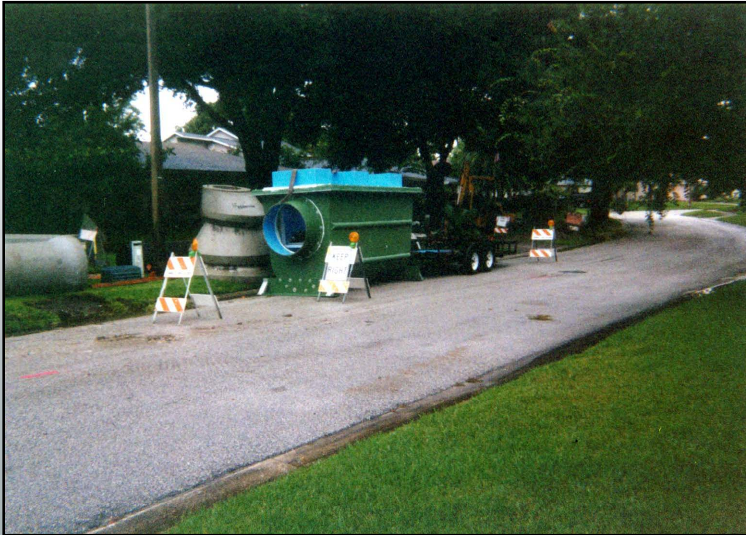
Photos of installation
