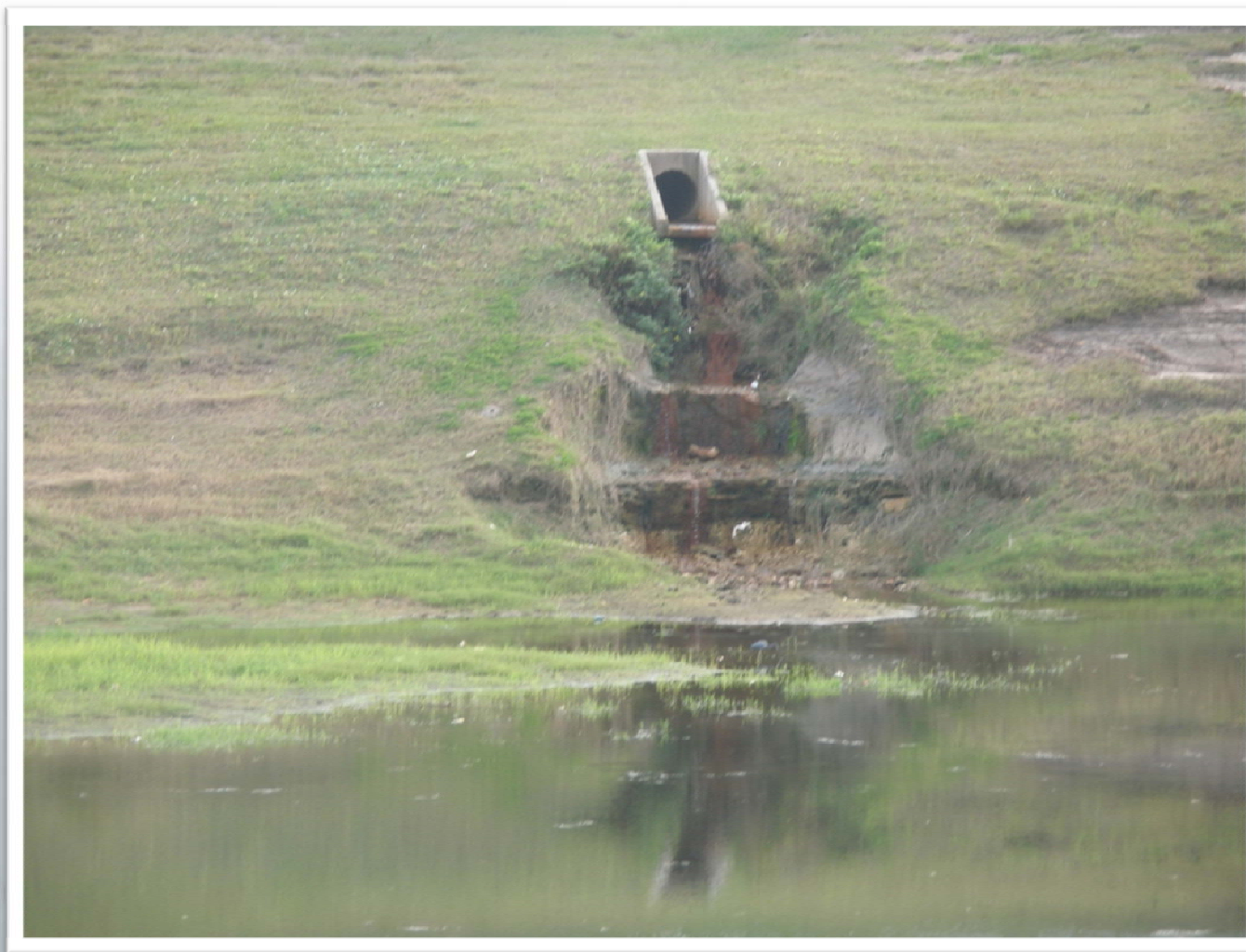
WESTLAKE-Resulting Cascading Outfall to Pond
