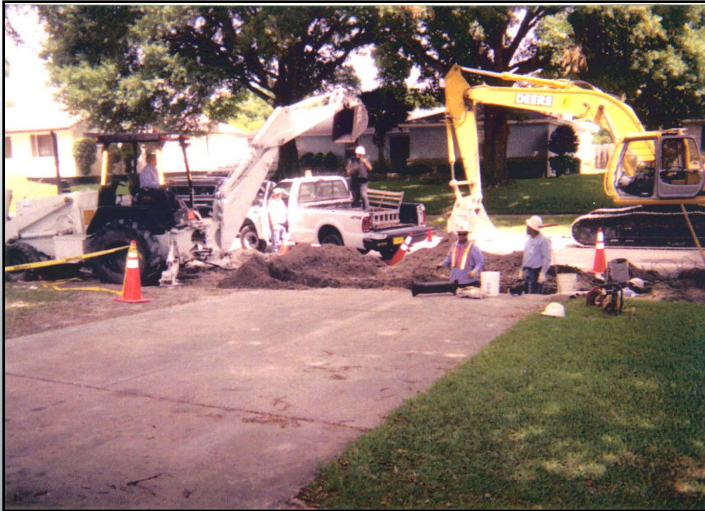
Photos of installation
