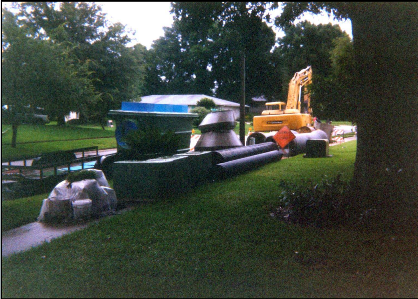
Photos of installation
