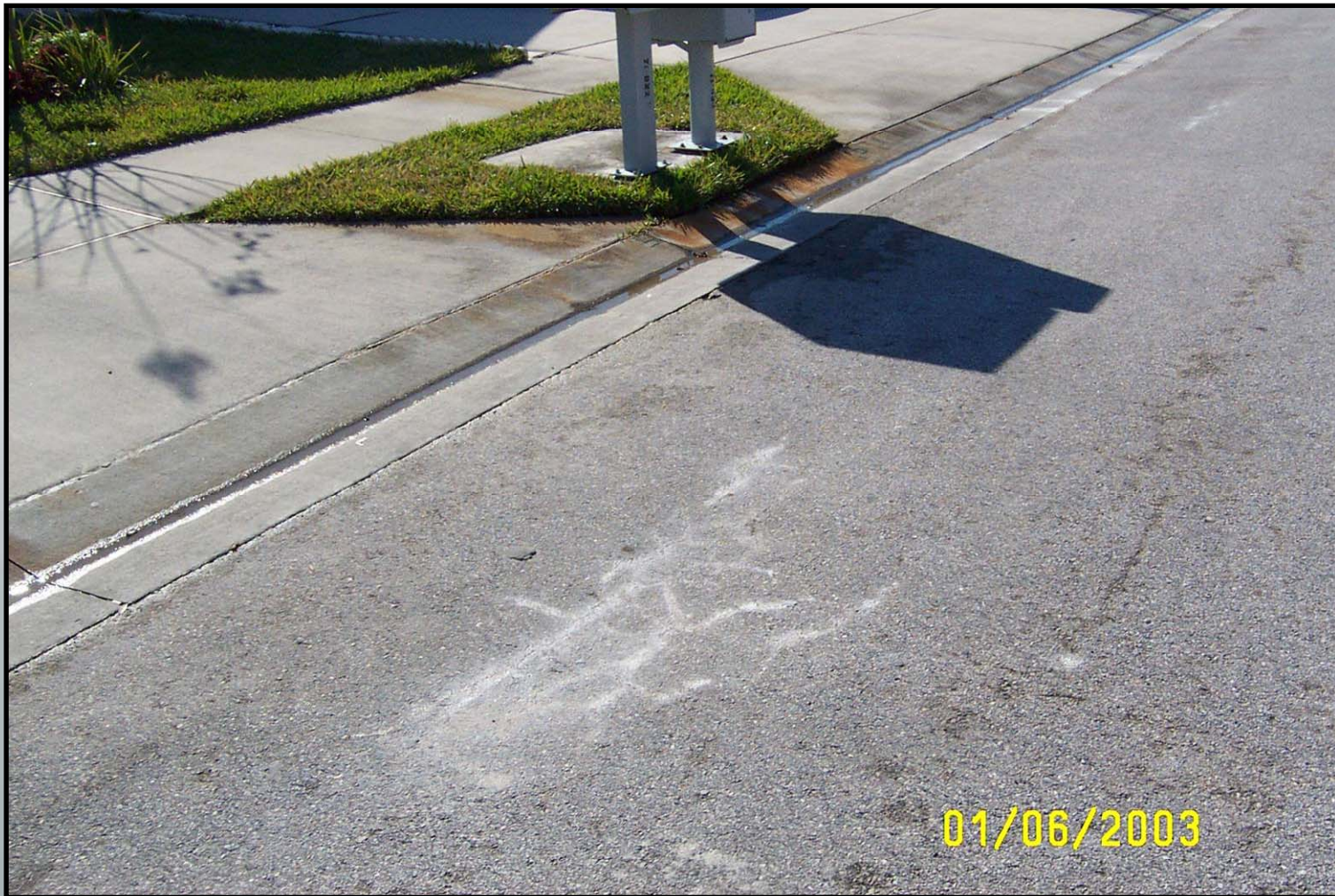
Limerock Pumping From Base
