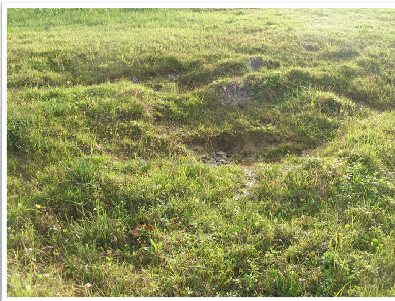
WESTLAKE-Seepage of Groundwater Resulting in Saturation and Sloughing of Slopes
