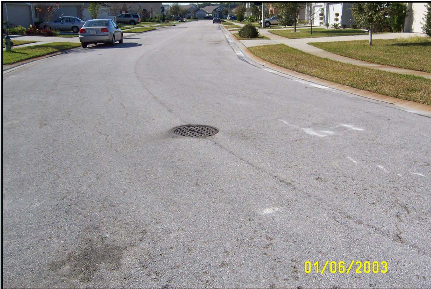
Limerock Pumping From Base
