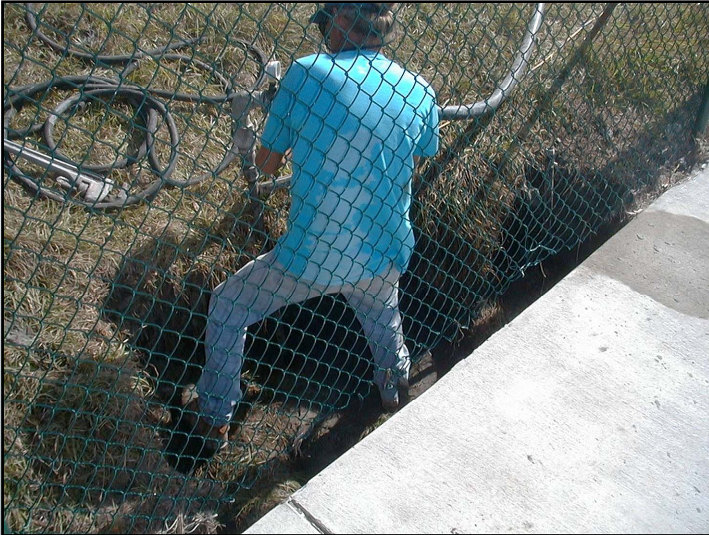
Grout being pumped into injection point
