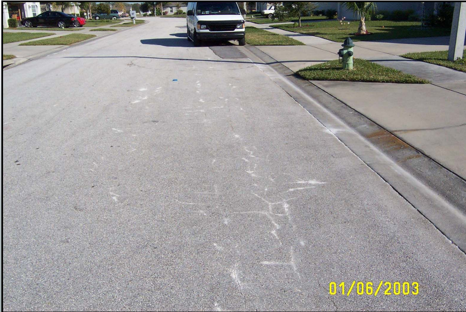
Limerock Pumping From Base
