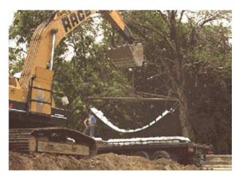
$\textbf{Figure TS14L-19} \qquad \text{Hand placement of ACB blocks}$
