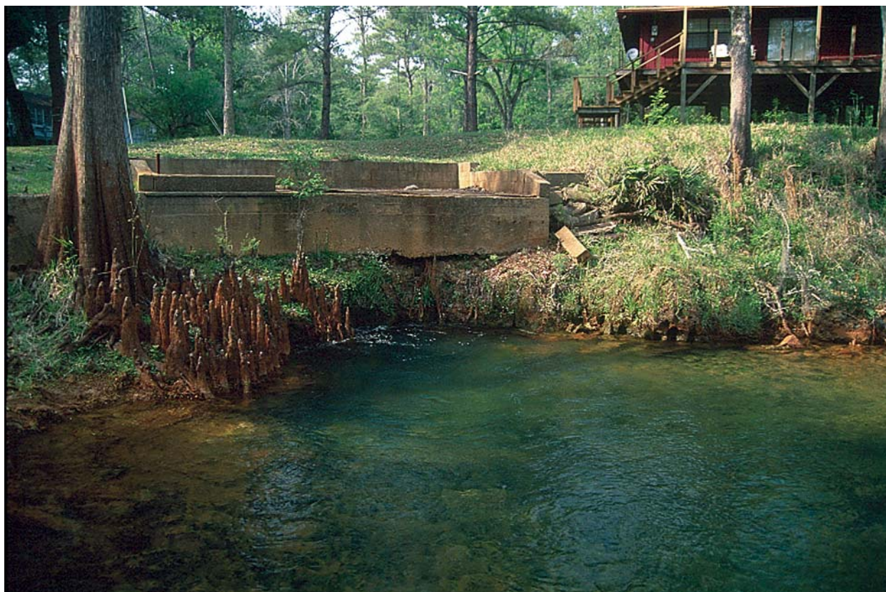
Figure 41. Copper Spring No. 2 (photo by R. Means).
