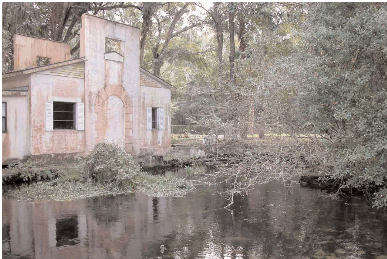
Figure 33a. Pumphouse Springs (photo by R. Meegan).
