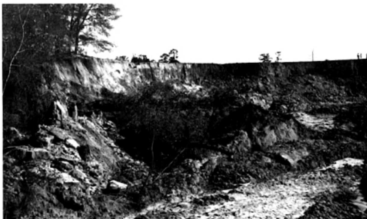
Figure 33. Photograph looking southwest at the scarp of the Pitt landslide. Note people at upper right. Photograph by R. O. Vernon, April 5, 1948 (Rupert, 1990).
