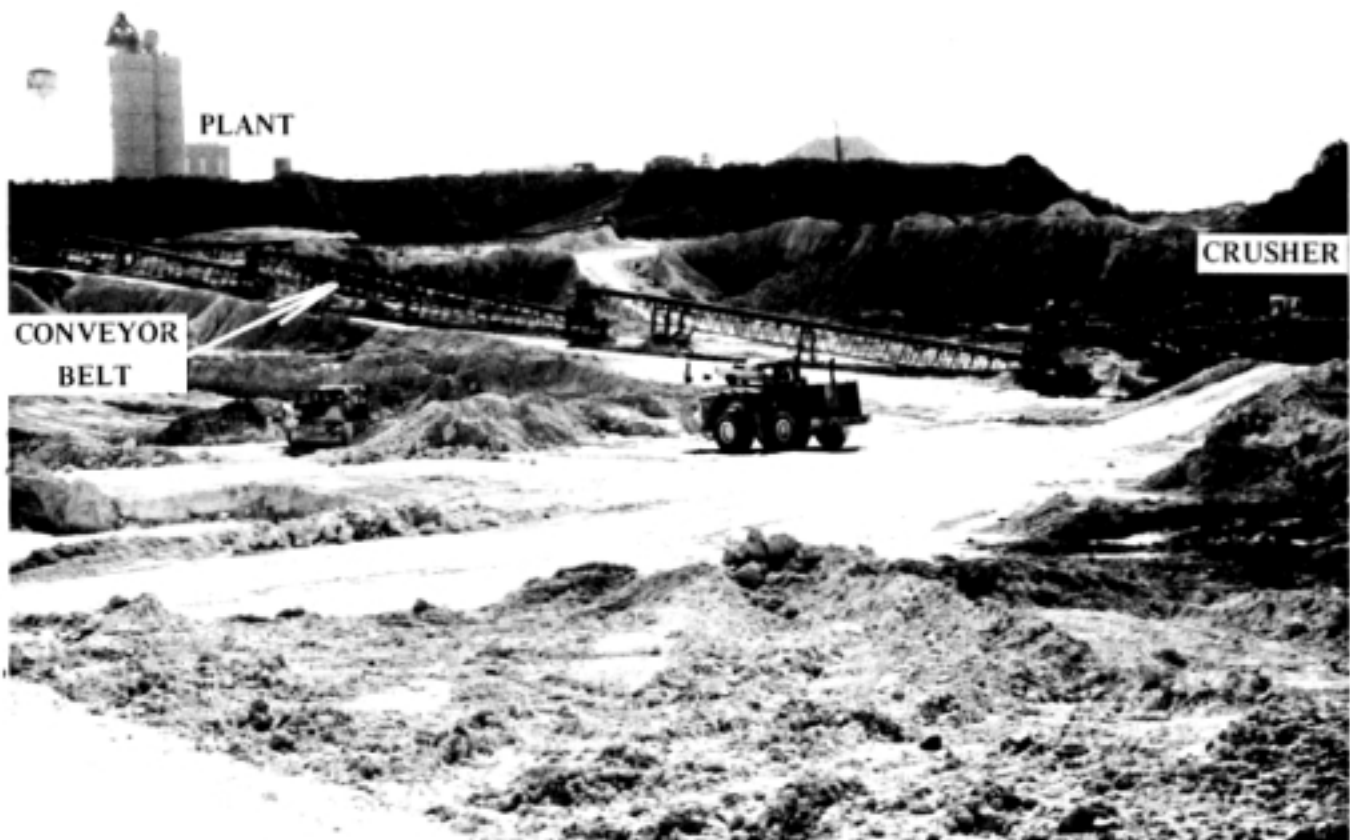
Figure 24. Open pit limestone quarry. Bulldozer rips and stacks rock; the front-end loader feeds the portable crusher; and the crushed rock is carried to the plant on the conveyor belt. FGS photograph.
