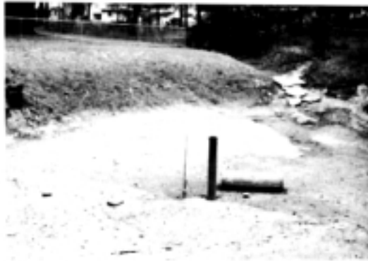
Drainage well in bottom of sinkhole carries storm water directly to aquifer (Lane and Hoenstine, 1991).
