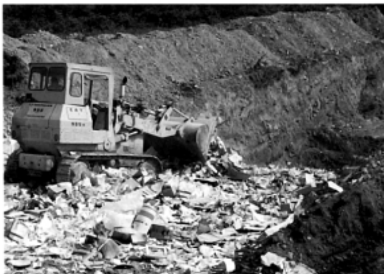
Figure 38. The old way of garbage and trash disposal: unsegregated refuse dumped in an unlined pit, compacted, covered with a few inches of dirt, and forgotten. Photograph by Ed Lane, 1968.
