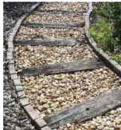
Recycled railroad ties, bricks and gravel make a unique footpath capable of absorbing rainwater.
