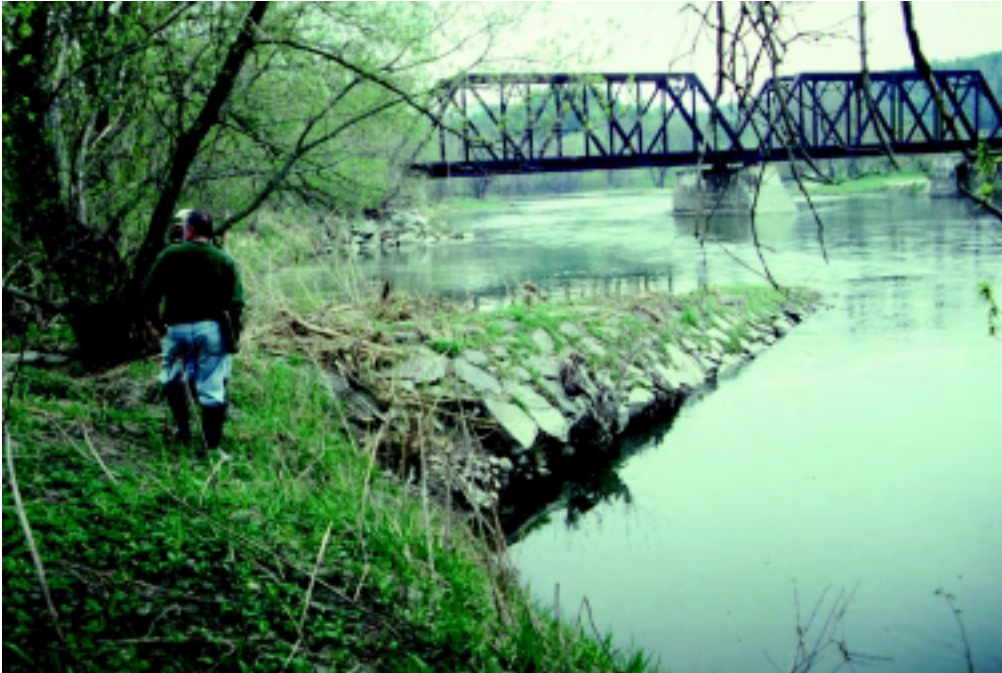
Figure 16-39a Stream jetty placed to protect railroad bridge
