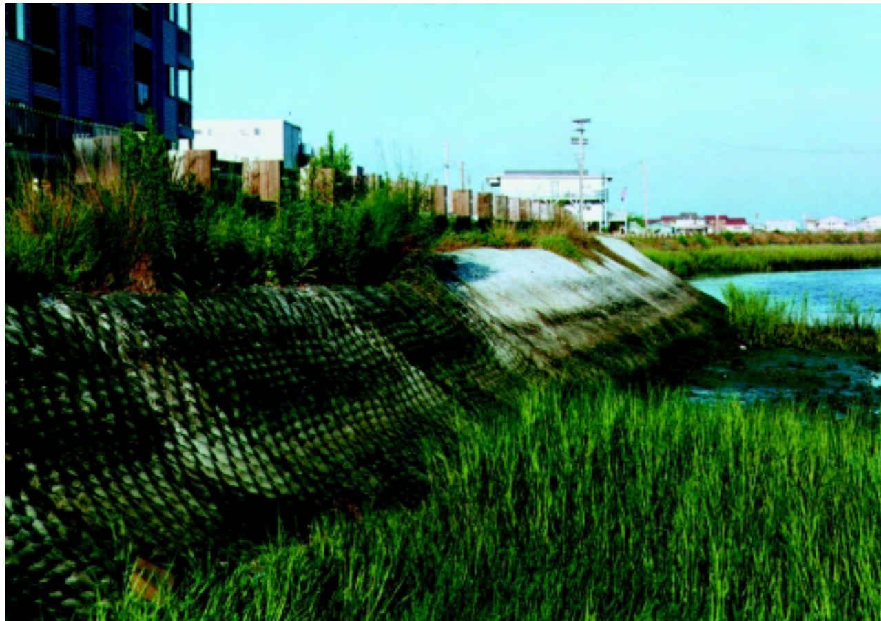
Figure 16-50 Concrete revetment (poured in place)
