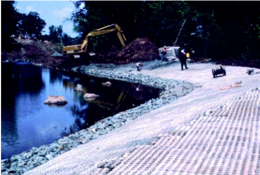
Figure 16-35a Concrete cellular block system before backfilling
