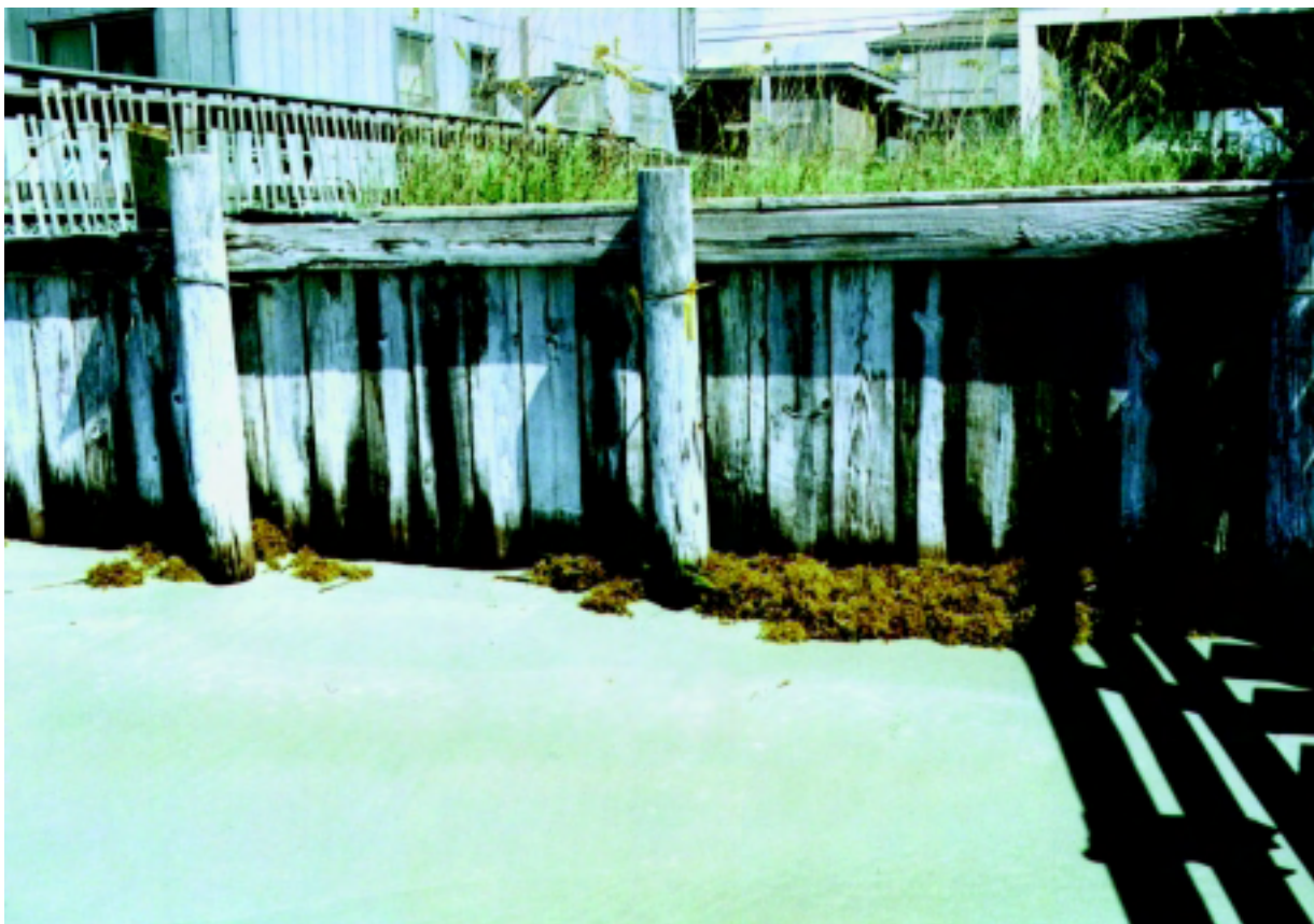
Figure 16-46 Timber bulkhead system
