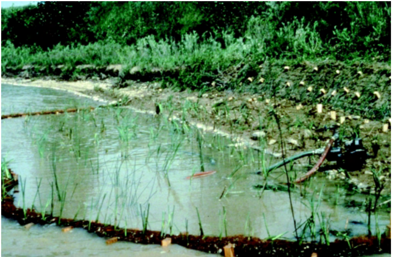
Figure 16-57 Coconut fiber roll system
