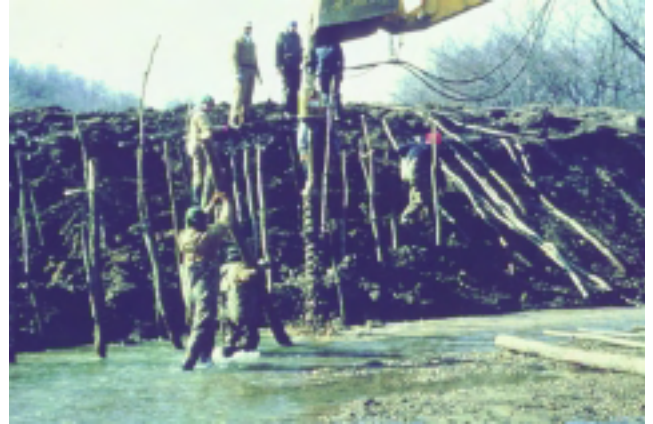
Figure 16-25b Installing dormant posts (Don Roseboom photo)
