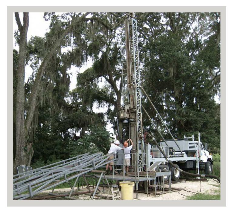
**Cover Photo:** Andrew Bowie and Barry Morley retrieve a rock core sample using the wire line on the UDR 200DLS core rig during exploratory coring at the ROMP 132 well site. Photo taken by Anna Janosik on August 3, 2010.
